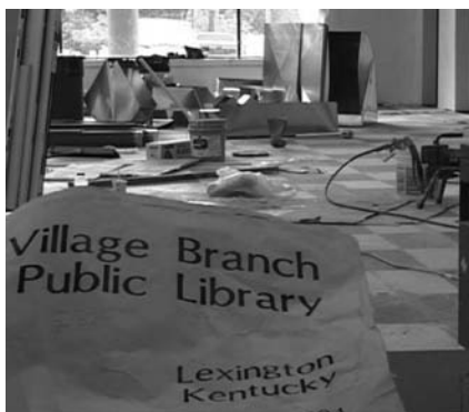
Figure 4: Beginning construction of Village Branch.
