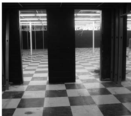
Figure 5: Village Branch prior to construction.
