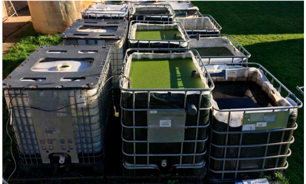
Figure 1. The three pilot-scale set-ups in which the influent is mixed and stored ( left ) before being pumped in the middle cubicontainer where duckweed is grown. With an overflow mechanism, the lower cubicontainer ( right ) is filled with effluent from the growing system.
