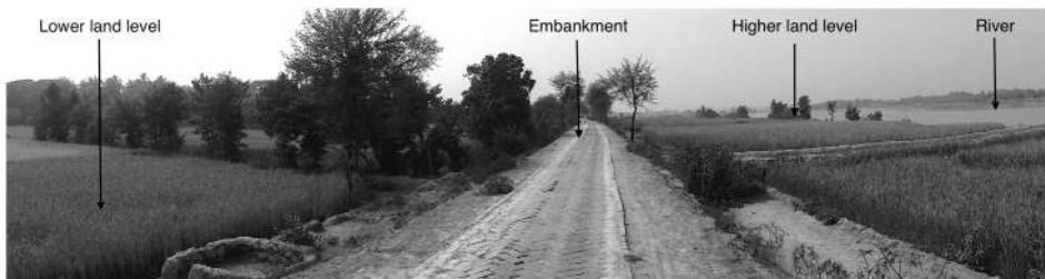
Figure 2. Embankment and raised banks due to siltation. Photo by Author.
