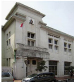
Figure 2. Gedung Gas Negara (PGN) Bandung, (Source: https://www.indischeliterairewandelingen.nl/ )
