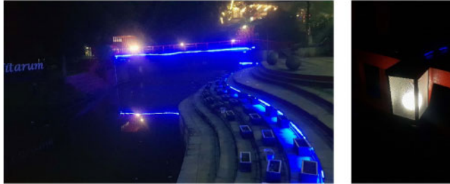
Figure 3. Perimeter illumination at the amphitheater and bridge at Teras Cikapunding in the form blue LED strip light, and bollard.
