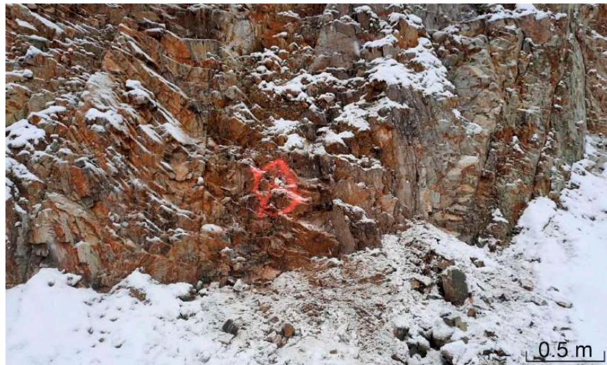
Figure 2. Weathered, strongly jointed granulite, corresponding to (2).
