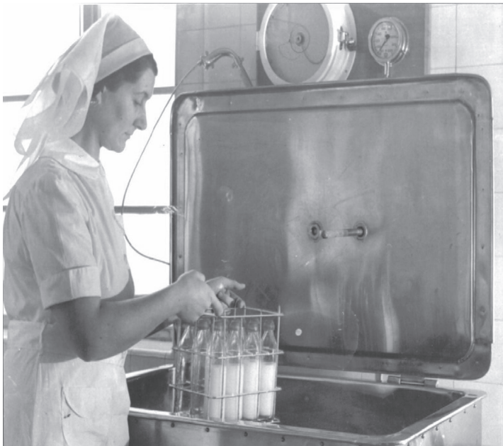
Figure 2.4 The bottles are placed in a basket which are then placed in the pasteurizing machine. Source: Reprinted with permission from Historic England.
