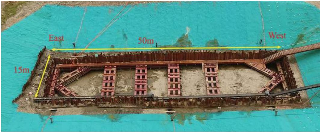
Fig. 10.4 Plan of sheet pile walls at the Jingtoushan site (Photo by G. P. Sun)
