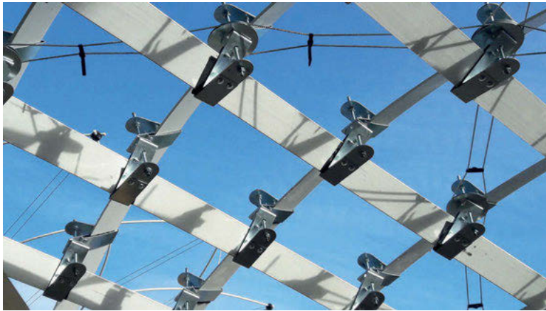
Fig. 9: The standard nodes developed in this study and bracing system. Laths cross-section: 100 × 8 mm.
