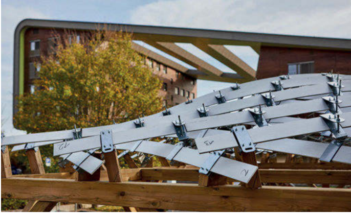
Fig. 4: The pseudo-geodesic pavilion, made of 100 mm GFRP lath at 60° with a unique Z-connector. (Picture: Charlene Yves)
