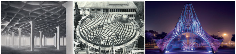
Fig. 1: Design practice inspired by PSL networks includes Gatti Wool Factory Floor System [8] (left), Zoology lecture hall at the University of Freiburg [9] (middle), and CIAB pavilion [13] (right).
