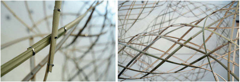
Fig. 7: Detail of the overlapping between bamboo slats (left); Connections occurring when cylinders start to shape nodes (right).
