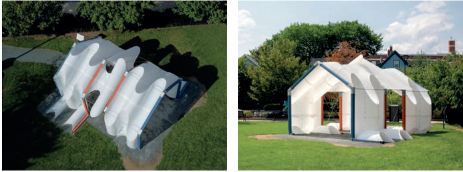
Fig. 4: Left: Aerial photograph of the shading pavilion. Right: The constructed prototype assumes the form of a gable in profile while containing a membrane surface that resembles a barrel vault.
