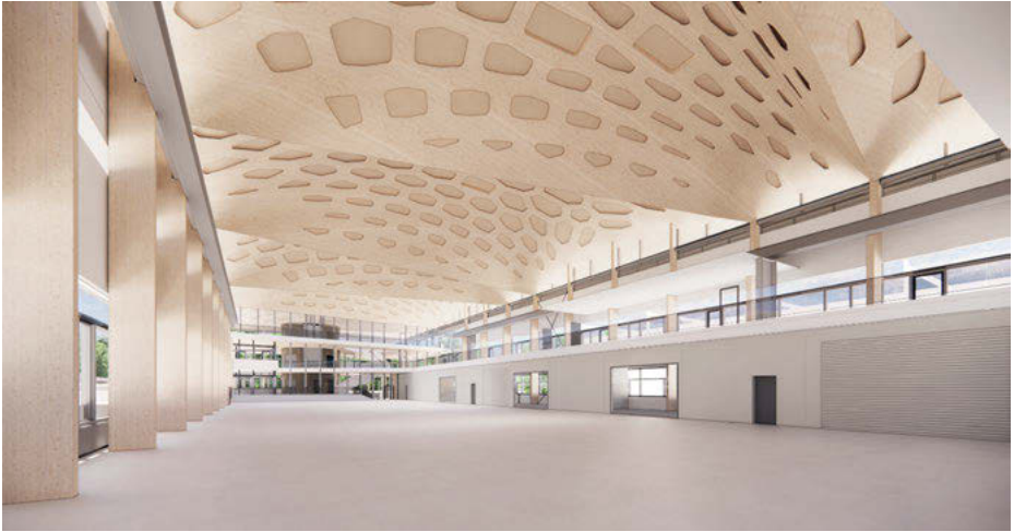
Fig. 9: Interior view of the LCRL hall covered by the segmented timber roof.
