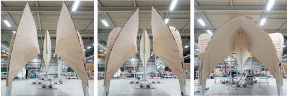
Fig. 5: In situ self-shaping of the bilayer timber building components. Starting flat in a vertical configuration with high MC in the active layer, during shaping, and after full shaping and interlocking.
