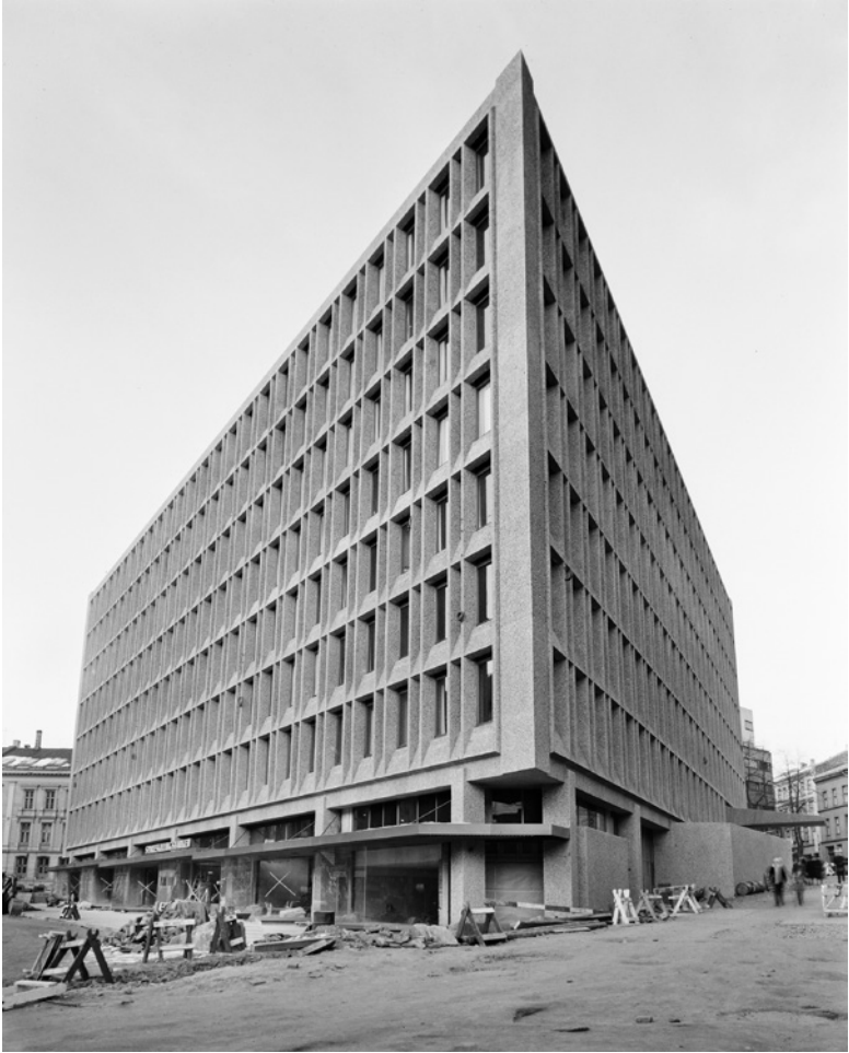
Figure 12.1 The Oslo Health Council anno 1969. The location posed several problems for the architects. The triangular shape was ‘not particularly well-suited for an office building’, the architects stated, and it had caused a range of technical and constructional problems. However, ‘the client saw a central location as the best solution’. Photo by Leif Ørnelund. With permission from the Oslo Museum, Creative Commons 3.0. http://www.oslobilder.no/OMU/OB.%C3%9869/0319 . Image available under a Creative Commons (CC BY-NC-ND 4.0) licence, https://creativecommons.org/licenses/by-nc-nd/4.0/ .
