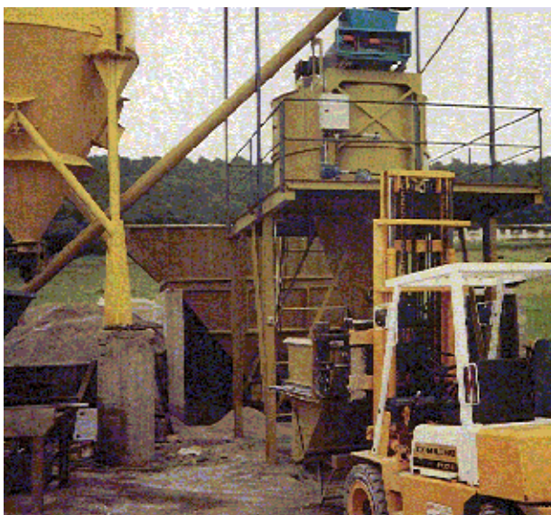
Fig. 5. The materials feeding and mixing platform
