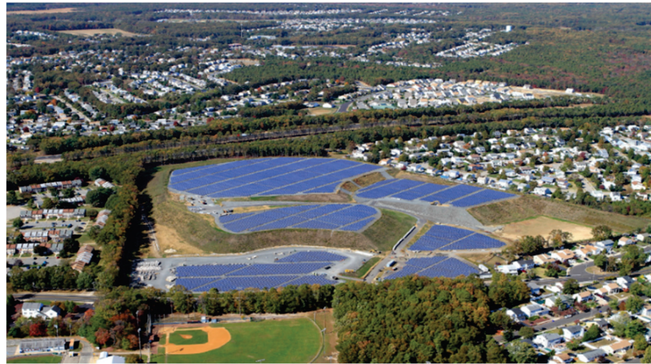
Figure 8. Brick Town landfill. Solar panel view [38].
