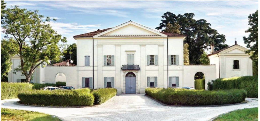
Figure 1. Villa Rivalta today. On the left, covered by trees, is Rota’s ancient annex building that is decorated with a pictorial cycle illustrating medical scenes.
