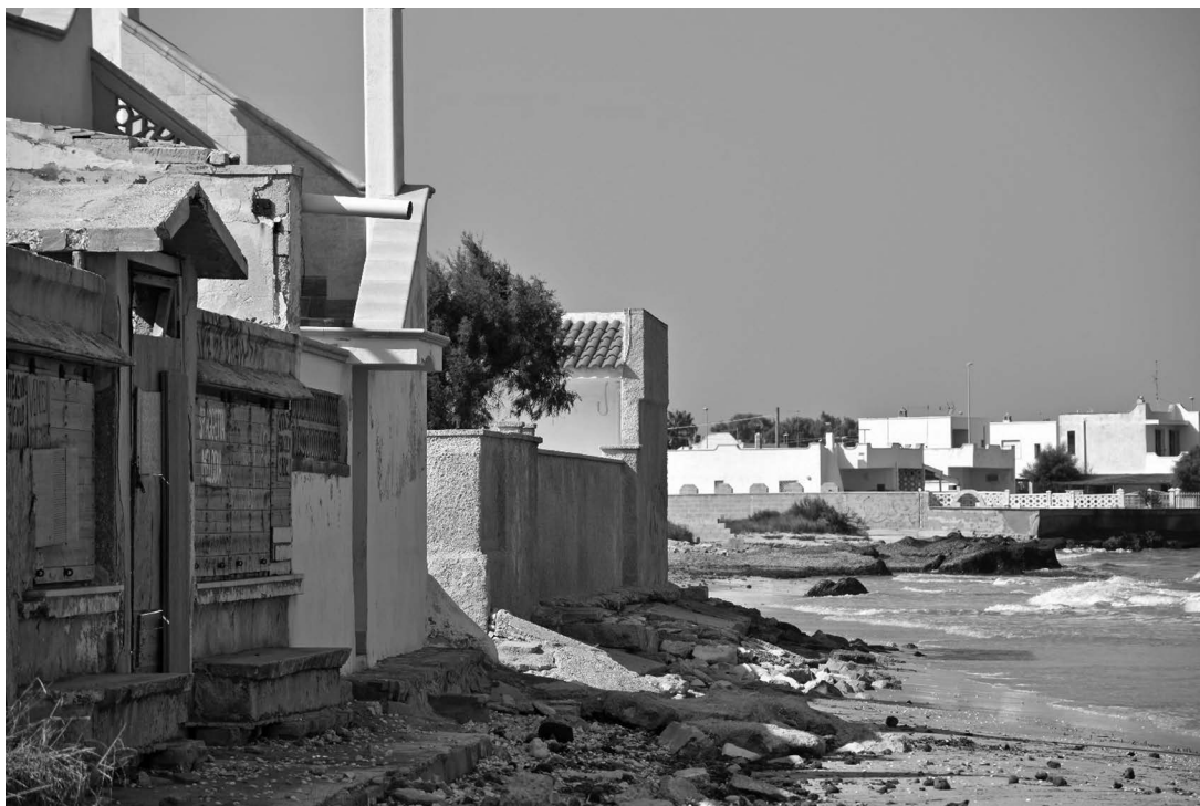
Figure 10.6 Illegal and legalized (after amnesty) buildings in the Lecce MPD
