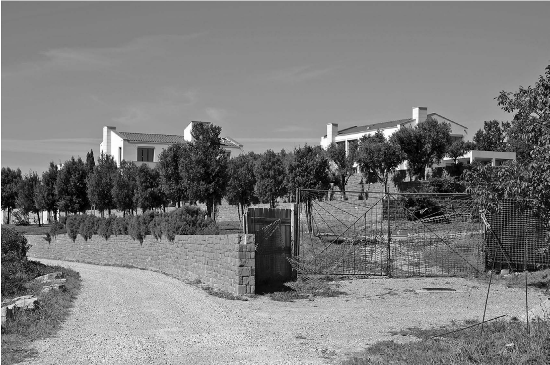
Figure 11.7 Half-built illegal tourist facility in Bužekija, Municipality of Izola
