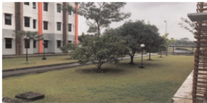
Figure 5. Façade area without ramp.
