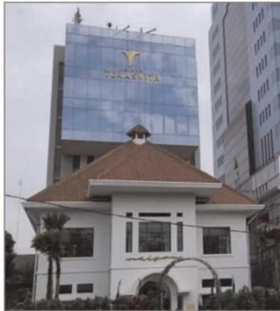
Figure 3. The old building (front) and the new building (back). Source: Beton Elemenindo Perkasa 2021.
