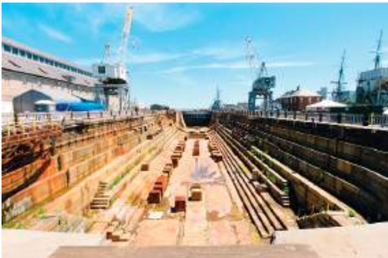
Plate 190 Graving dock showing bottom blocks. Any additional tasks that are undertaken while the dock water is being pumped out would also be noted in the log book, e.g. cleaning and scrubbing around the hull by work punts in the area of the waterline as the level falls. (Source: Shutterstock.)
