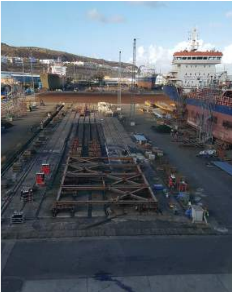
Plate 188 Tracked docking bay seen with exposed ship carriage, at the synchro-lift docking park in Las Palmas, Canary Isles.
