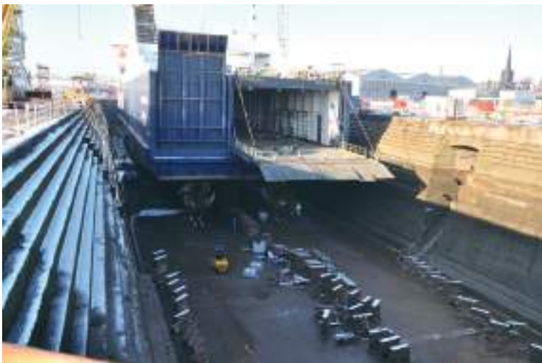
Plate 194 On the blocks in a graving drydock. A ro-ro vessel seen from astern with its stern door/vehicle ramp open. Spare keel and bilge blocks are seen on the floor of the dock.
