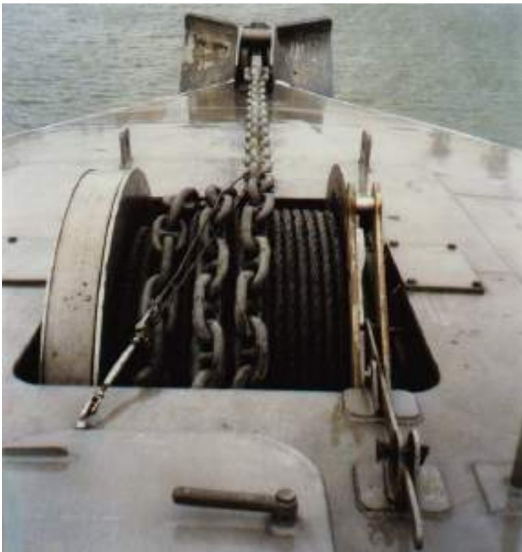
Plate 19 Single centreline anchor arrangement in the bow of a high-speed craft ferry. Use of combination short chain cable and anchor warp is to reduce carriage weight of all chain.
