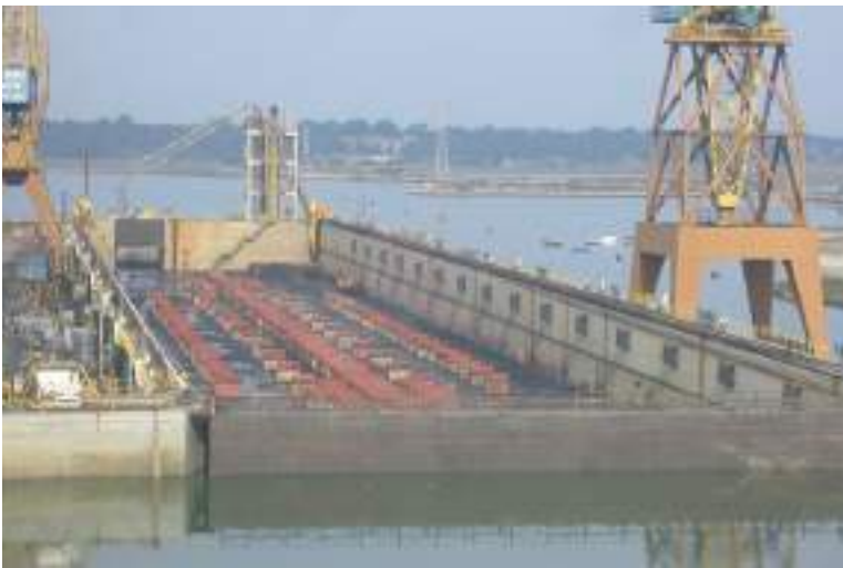
Plate 193 The 'block pattern' spread in the Hydrolift dry dock at Lisnave, Portugal, ready to receive the next vessel. Information from the drydock plan allows the blocks to be placed in the correct order to take the ship without causing damage to the vessels appendages.
