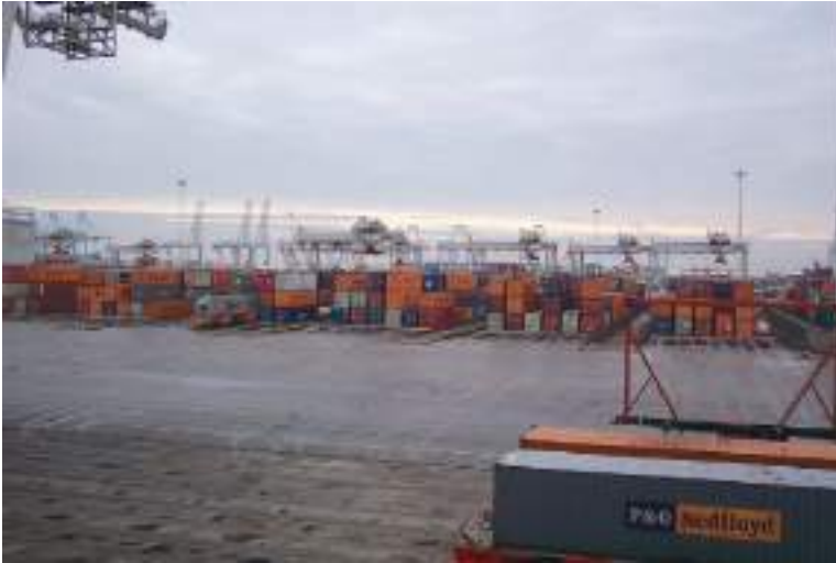
Plate 67 Shoreside container terminal park in Japan, showing container stacks and travelling overhead carriage cranes. Container movement from the park to the ship loading gantries is by driverless ground handling transports.
