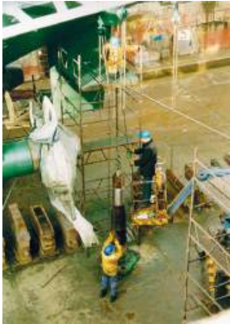
Plate 195 Typical drydock operation where the rudder post is withdrawn for inspection.
