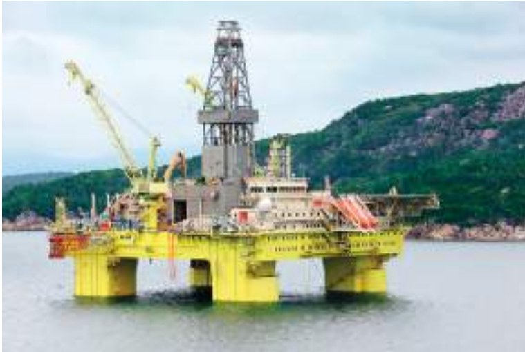
Plate 175 Offshore fixed installation. (Source: Shutterstock.)
