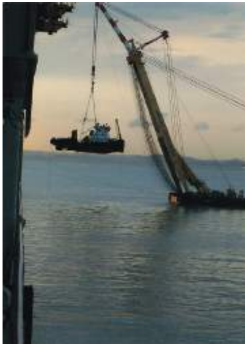
Plate 27 Heavy lift being made by floating sheer legs.
