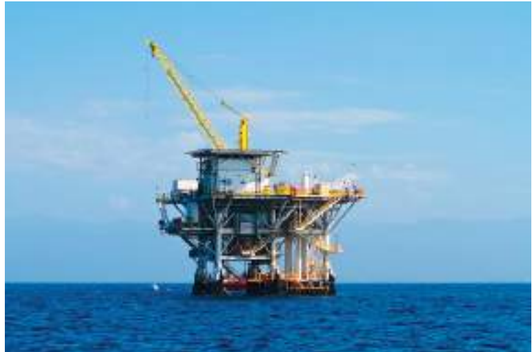
Plate 173 Operational offshore installation. (Source: Shutterstock.)
