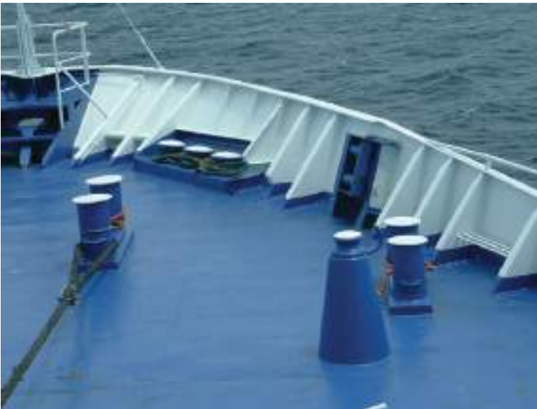
Plate 238 Forward mooring deck of a passenger vessel, showing triple roller fairlead on the starboard bow. A universal roller lead inset on the starboard side and two sets of bitts (bollards) seen forward of an 'old man', roller lead.
