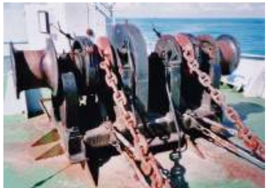
Plate 14 Centreline windlass. Cables seen are secured by devil's claws and wire/bottle screw lashings.
