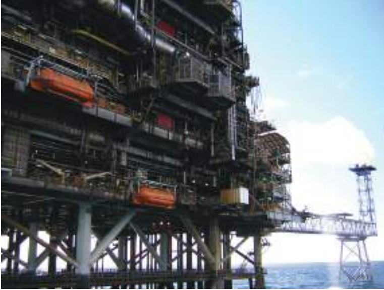
Plate 78 Totally enclosed lifeboats seen in situ on an offshore installation.
