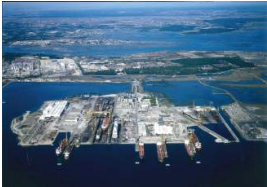
Plate 189 The Lisnave shipyard, Portugal. The wet basin and the three docking platforms are seen in the Hydrolift complex to the right of the overhead view.
