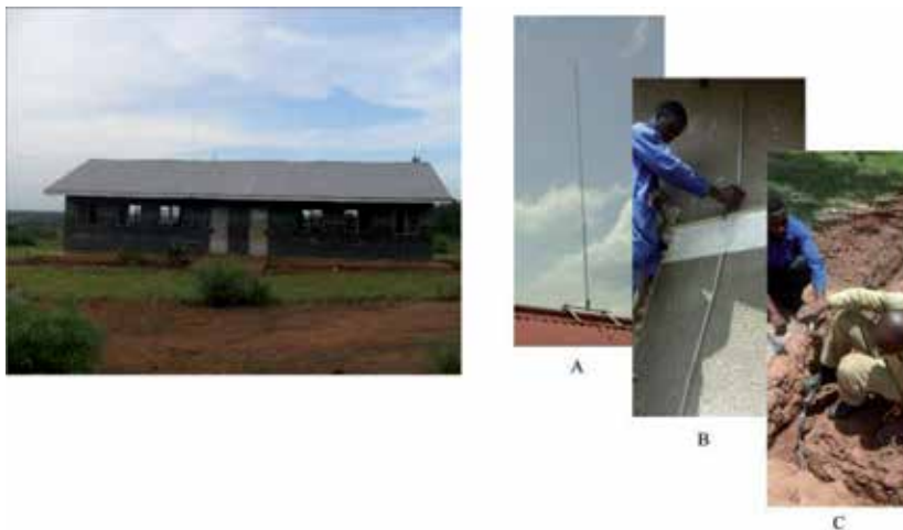
Figure 10. Installation of lightning protection system at a typical classroom building at Runyanya school, Uganda. Details: (A) air terminal; (B) down conductor; and (C) ground terminal or "earthing ring." (©ACLENet).
