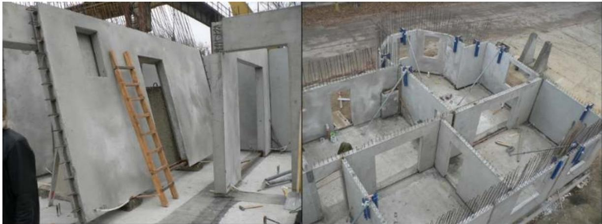
**Figure 6.** Prototype of prefabricated house IDA I—view of the innovative panels with built-in thermal barrier and construction of the first floor [1].
