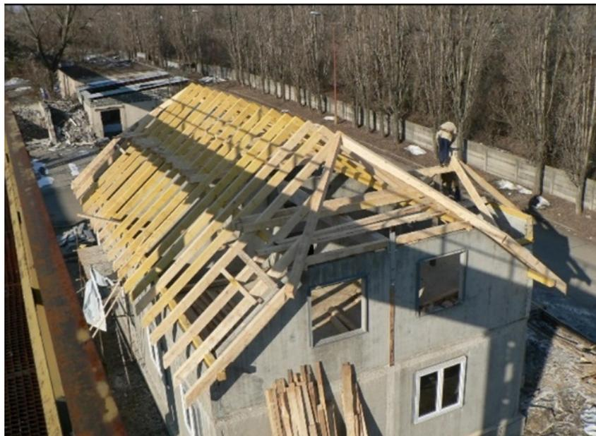
**Figure 29.** View of the realization of the wooden truss (photo archive: Kalús, D.) [1].
