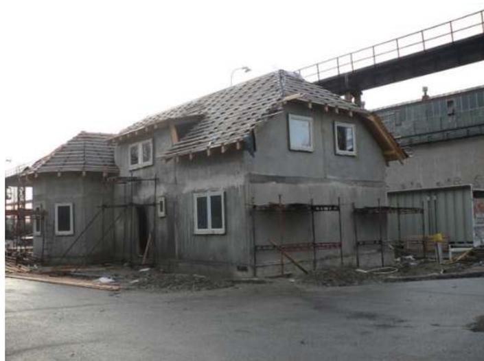
**Figure 1.** A view of the construction of the prototype prefabricated house IDA I [1].
