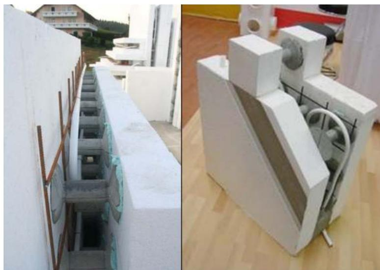
**Figure 3.** View of the lost formwork of the ISOMAX panel and the principal location of the thermal barrier [2].
