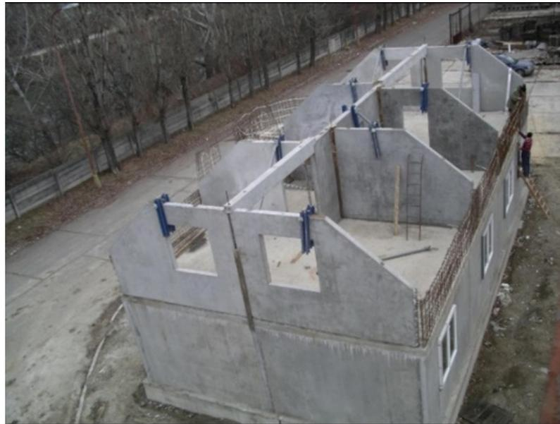
**Figure 28.** Completion of the ground floor assembly (photo archive: Kalús, D.) [1].
