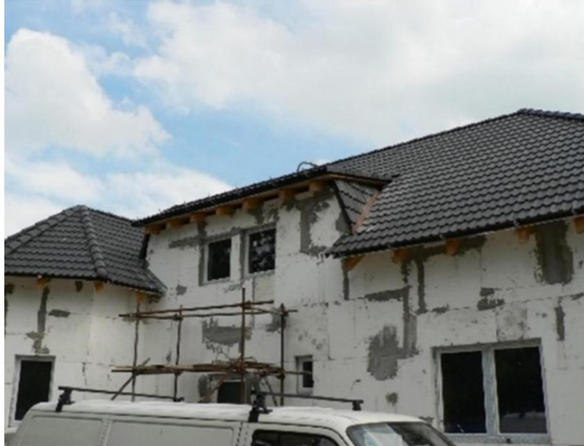
**Figure 30.** View of the implementation of the insulation of the perimeter panels (photo archive: Kalús, D.) [1].
