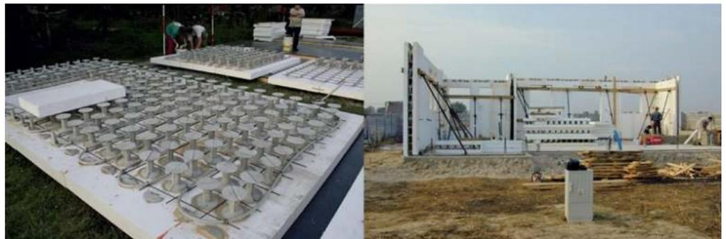
**Figure 2.** View of ISOMAX panel production from lost formwork [2].
