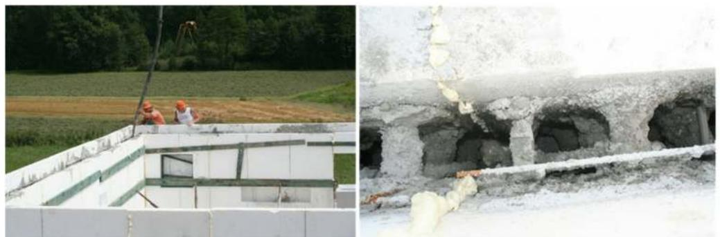
**Figure 17.** Construction with patented ISOMAX panels [2].
