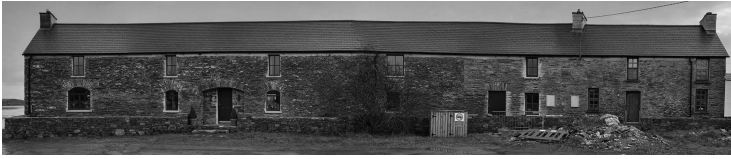
Figure 7.5 Composite elevation of former warehouse building on Quay from rectified photographs by Canty and Eckardt 2021, with modelling by Julianna O'Donoghue 2022.
