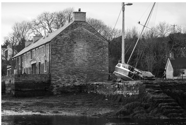
Figure 7.7 The original pitch line of the roof of the warehouse and the outline of the crane door can be discerned. Photograph by Kevin O'Farrell 2021.
