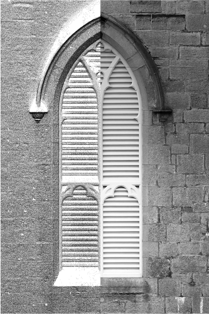
Figure 5.5 Elevation of a window of a church: Point cloud image to the left, Photomosaic image to the right. Image reproduced with permission from Geomap.
