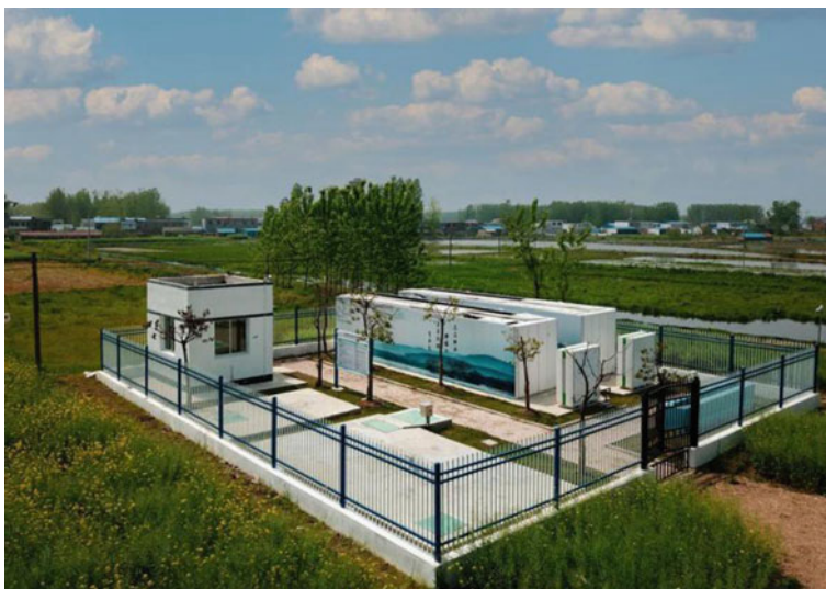
Fig. 5.12 The site of a rural domestic sewage treatment case in Huangshan, Anhui, China
