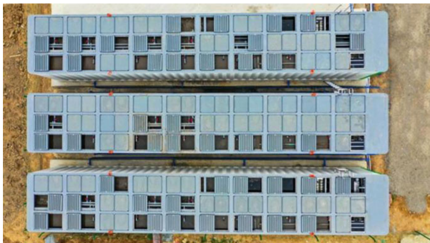
Fig. 5.20 Site of A domestic sewage treatment case on campus in Haikou, Hainan, China
