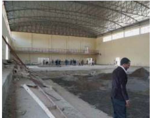
The gymnasium of Arsi University under construction
