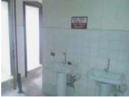
The toilets just before the renovation was finished
