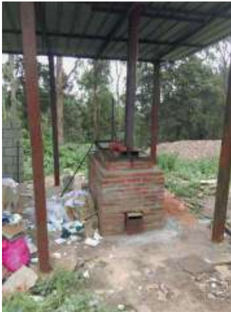
The newly-built incinerator in June 2016
