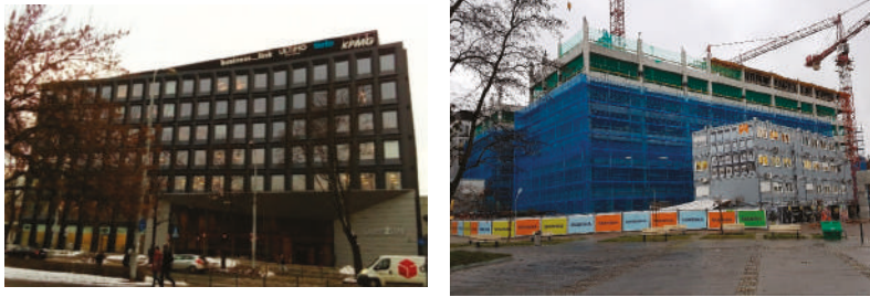
Figure 2. “Green2Day” office building front view. Investor: Tenali Investments Ltd. and Trikala SCA. Designers: Maćków Pracownia Projektowa LP & Grupa Projektowa Konstruktor Ltd. Own study.
