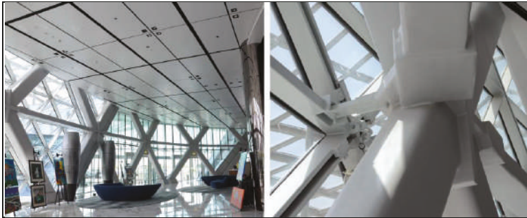
Figure 20. Capital Gate Tower: Diagrid structure—view from the interior (photograph by authors).
