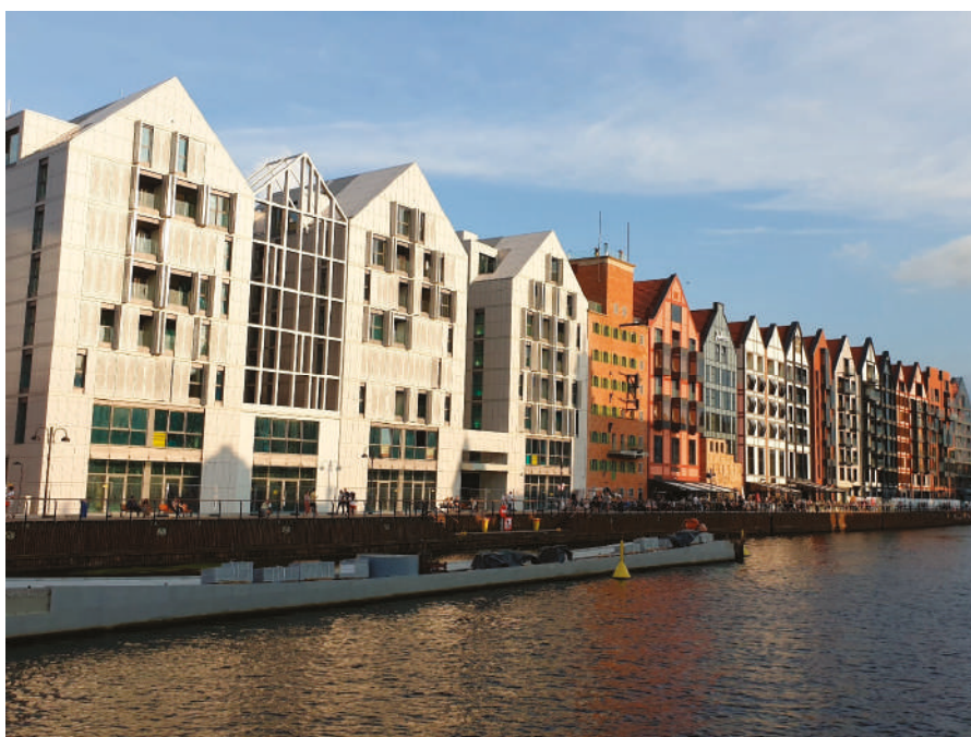
Figure 6. Gdańsk—modern facades on the banks of the River Motława (photo by J. Tymkiewicz).
