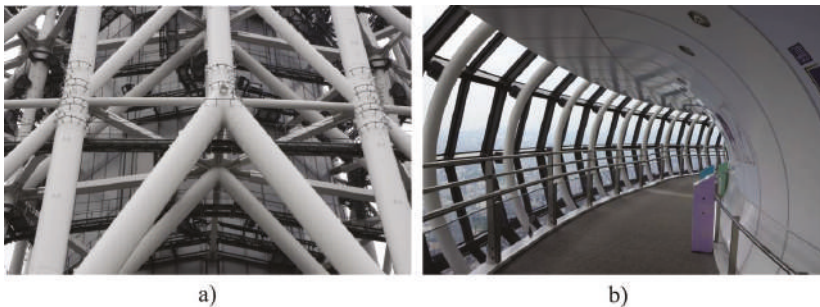
Figure 17. Tokyo Sky Tree: (a) An independent steel truss structure employing wide-bore high strength steel pipes; and (b) the spiral ramp of the Tembo Gallery in the second observation deck (photograph by authors).
