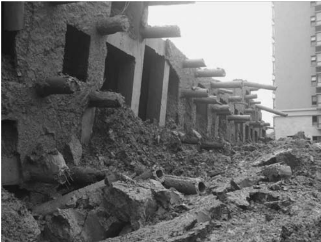
Figure 2.6 Detail of the foundation piles (Internet photo).
