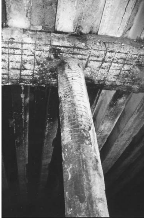
Figure 5.18 Concrete cover pushed off at larger areas due to thermal incompatibility between concrete and steel cage.
