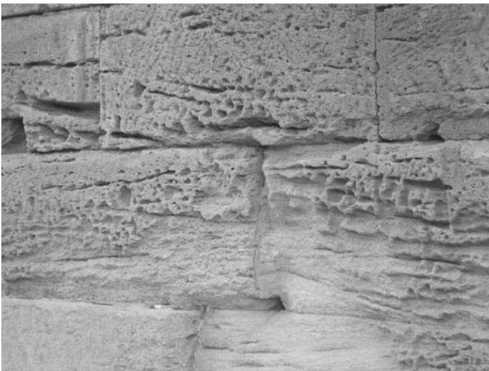
Figure 1.2 Pont du Gard, France, degradation of the limestone.
