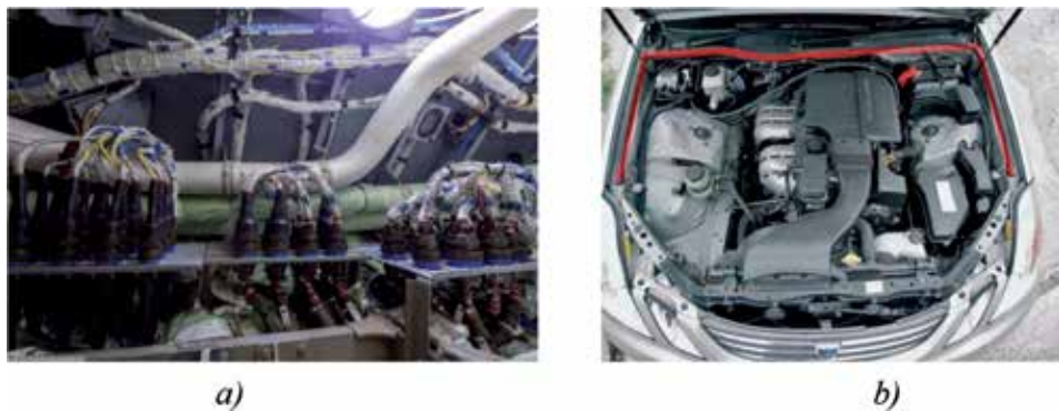
Figure 15. An example of laying the trace: (a) electric furnace and (b) the air duct channel of the car.
