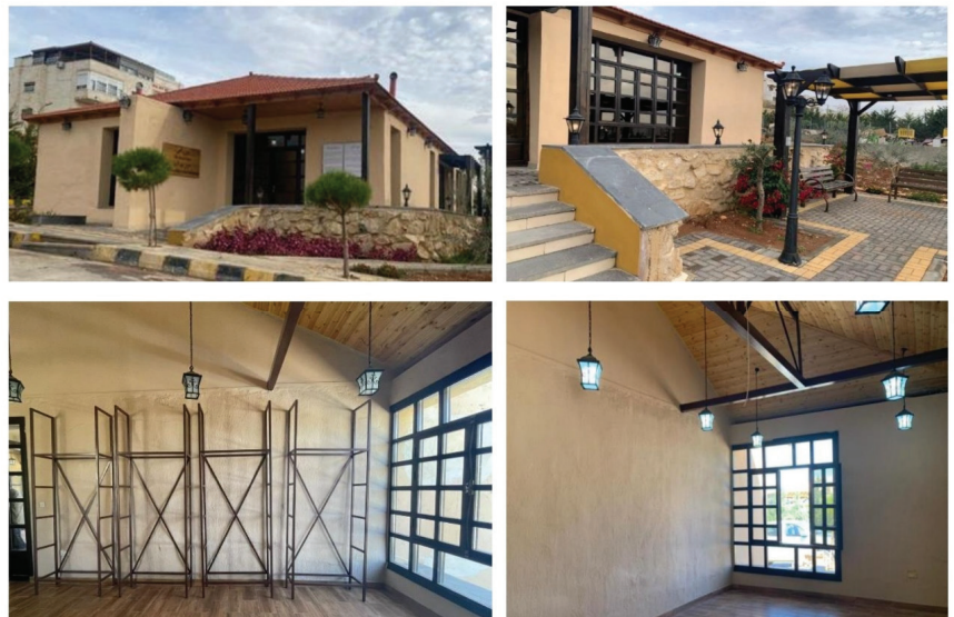
Figure 11. External and internal views of the constructed rammed earth building.
