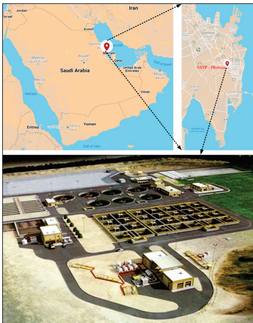
Figure 1. Geographic location and an aerial view of the Dhahran North Sewage Wastewater Treatment Plant (DWWTP).
