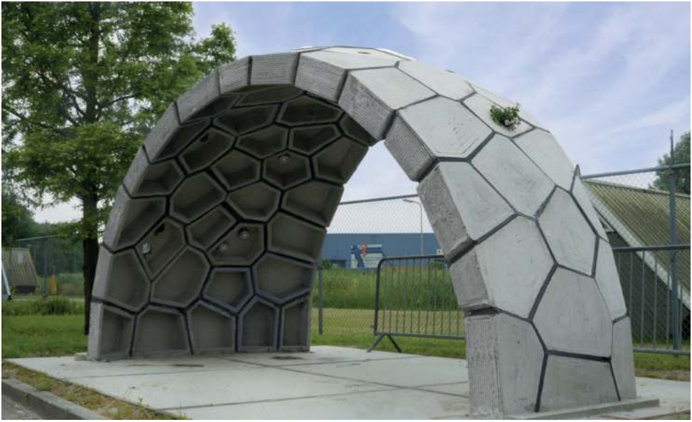
Figure 4 Green Dome Case, 3D concrete printing and para- metric design.
