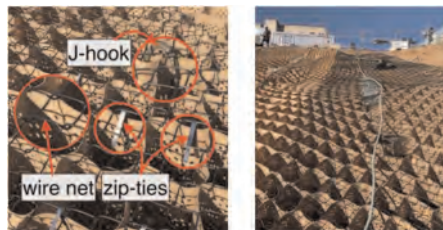
Figure 5. Installation of wire net with geocell.
