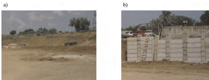
Figure 7. The initial and final stages of the landslide protection structure construction during the 2013 summer in the area of the Vertolit Research Center boathouses location (Prymorske village, Feodosia, Autonomous Republic of Crimea, Ukraine): a) – natural slope: b) undercut slope fixed according to the project. The planned monitoring of the reinforced wall was not carried out due to the annexation of Crimea by the Russian Federation in the spring of 2014.
