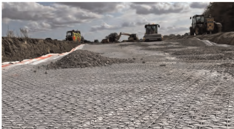
Figure 9. Installation of the pavement capping layer at North Heybridge (Tensar International Ltd).
