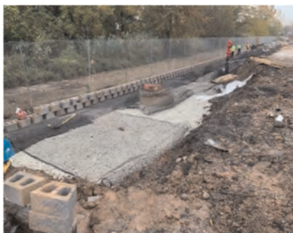
Figure 3. Photo of AASHTO #57 installation.
