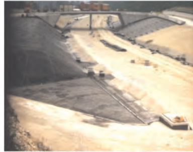
Figure 7b. Exit covered by BGM.
