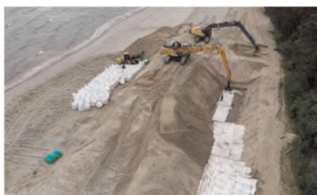
Figure 14. Installation of Geotextile Sand Containers as coastal protection measure in the dune core of the sandy beach, Ludmin Germany.
