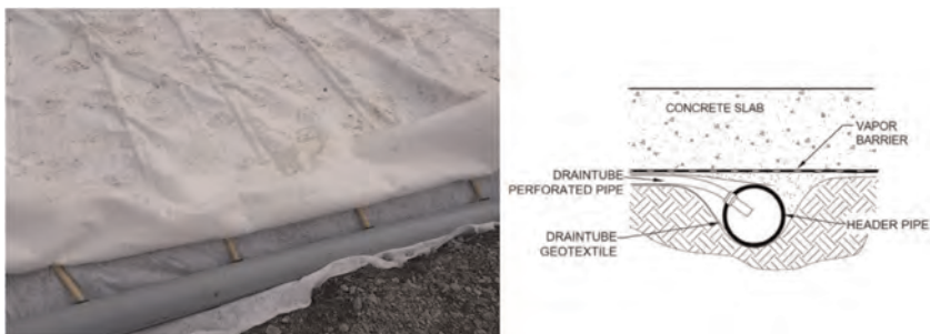
Figure 3. Connection to the header pipe.
