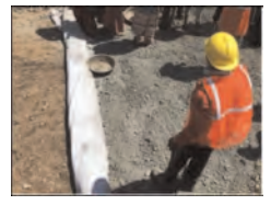
Figure 10. Infilling 100mm thick blanket layer.
