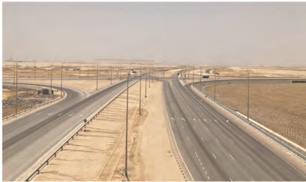
Figure 11. Roads completed in Duqm on basal reinforced embankments.
