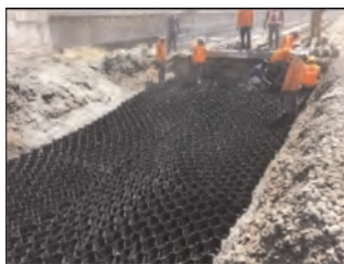
Figure 12. Bottom-most geocell layer.
