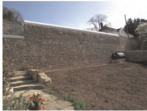
Figure 3. Finished wall with masonry reattached.
