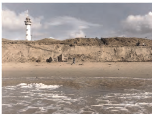
Figure 2. Severe dune erosion after storm surge, Egmond aan Zee lighthouse, The Netherlands.
