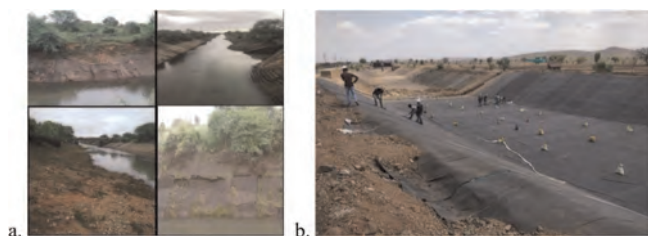
Figure 9. a. Irrigation canals in India – before / 9.b. Irrigation canals in India – during installation.
