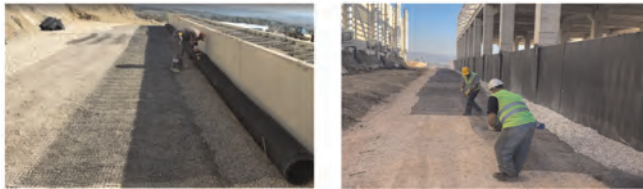
Figure 5. Installation of geogrids.
