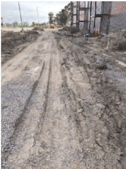
Figure 3. Installing crushed rock capping layer over geogrid.
