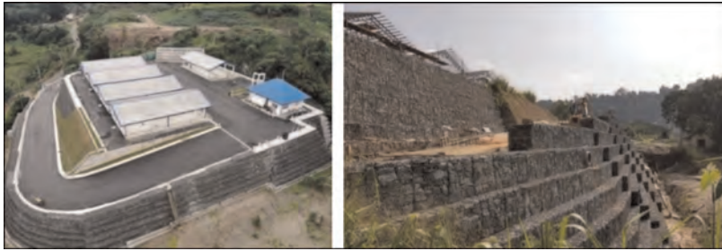
Figure 7. Completion of reinforced soil retaining slope.
