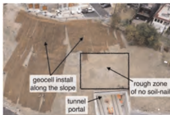
Figure 4. Layout of the slope with tunnel portal.
