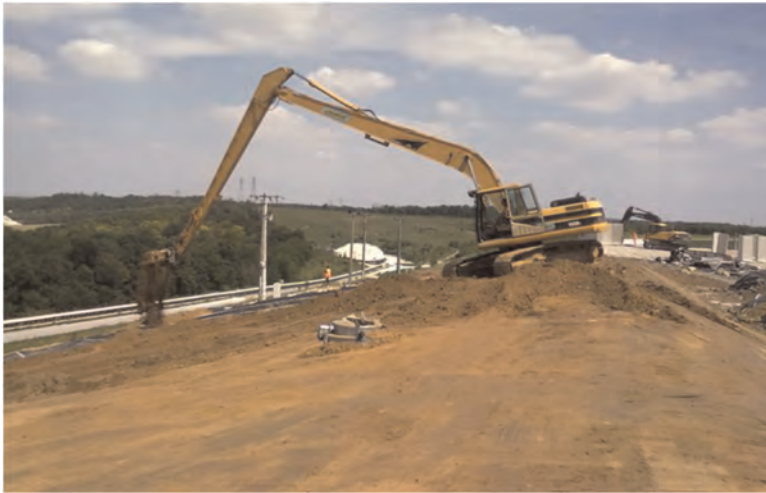
Figure 3. Long arm shovel able to work at over 20 m.
