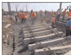
Figure 16. Placing sleepers over ballast.
