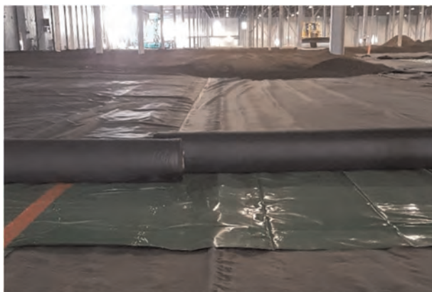
Figure 4. Vapor barrier and geotextile installation.
