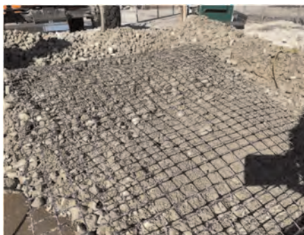
Figure 2. Close-up of UL-FGA and geogrid.
