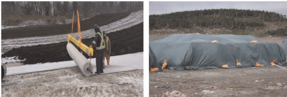
Figure 1. Winter deployment and GCL rolls being stored over the winter until deployment. A GCL made with a dry bentonite can be stored without any concern over the winter season outside until required for deployment.
