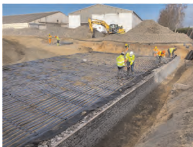
Figure 2. Installation phase of ParaLink geogrids ® in combination with Terramesh Systems ® .
