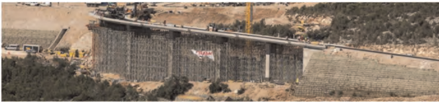
Figure 5. Replacement of external portions of the Brijesta viaduct with reinforced earth embankments (total length about 200 m, maximum height about 15 m).
