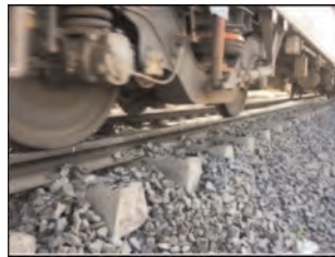
Figure 20. Finished track surface at the bridge - approach transition zone.
