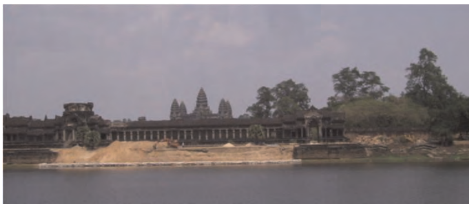
Figure 1. Intervention area during the rehabilitation intervention.
