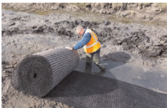
Figure 15. Installation of a reinforced High Performance Turf Reinforcement Mat (HPTRM) for slope protection.
