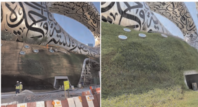
Figure 8. Green Terramesh reinforced soil structure: before and after vegetation growth.
