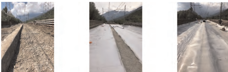
Figures 1 – 2 – 3 Typical application phases on site.
