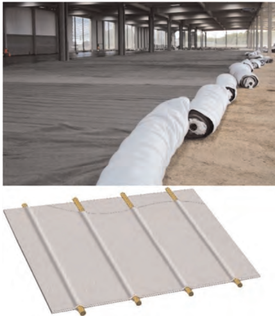
Figure 2. Installation of the geocomposite on the subgrade.
