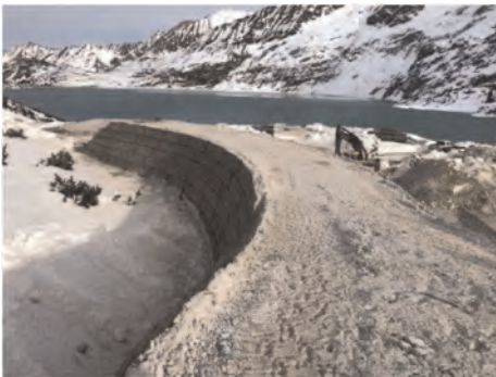
Figure 2. Tauernmoos avalanche deflecting dam during construction. (Nov. 2021).
