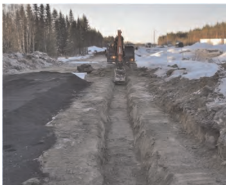
Figure 4. Excavation of trench.
