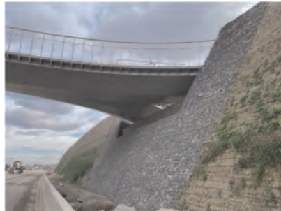
Figure 3. Reinforced soil structure made with Terramesh Green ® and Terramesh Mineral ® units underneath a cycle bridge overpass.
