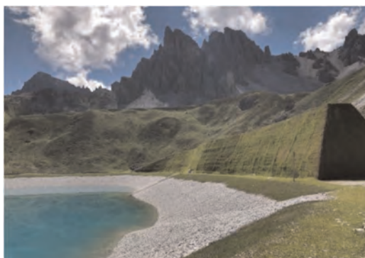
Figure 4. Avalanche protection dam Axamer Lizum after completion.
