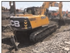
Figure 5. Removal of sleepers.
