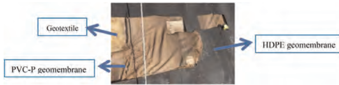
Figure 3. Appearance of the PVC-P geomembrane under the HDPE geomembrane in the crest area of the north slope at 216 months.
