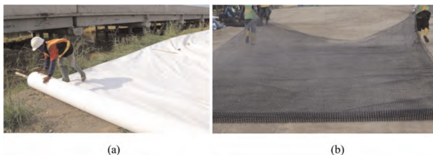
Figure 2. (a) Non-Woven and (b) Geogrid.
