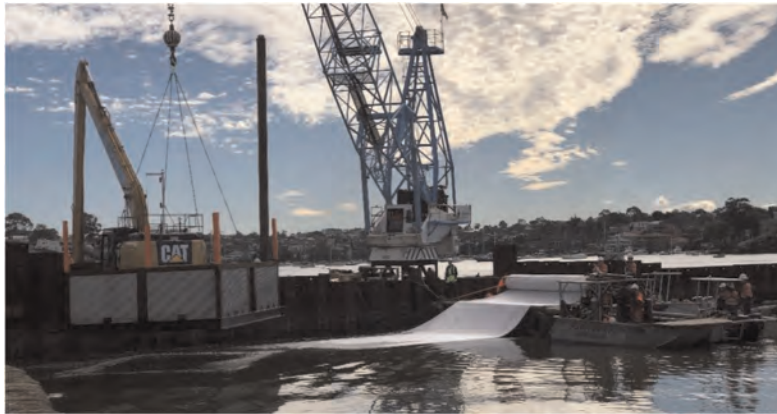
Figure 4. Installation of active geocomposite with bottomless frame (Courtesy of HUESKER Australia).
