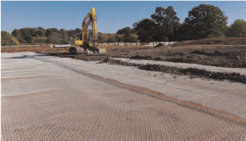
Figure 8. Installation of the working platform at HS2 Stoneleigh Park (Tensar International Ltd).
