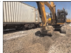
Figure 6. Removal of ballast.
