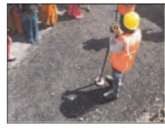
Figure 11. Compaction with manual hand tamper.
