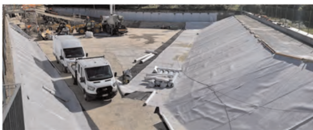
Figure 8. Photo of the geocomposite placing activities.
