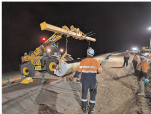
Figure 2. Innovative High Friction Angle (HFA) BGMs being deployed on slopes for mine waste capping and environmental protection. Northern Territory, Australia.
