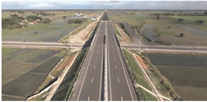
Figure 6. The CLLEx completed with pavement constructed on top of the reinforced embankment.
