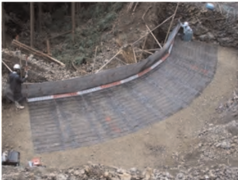
(a) During construction
