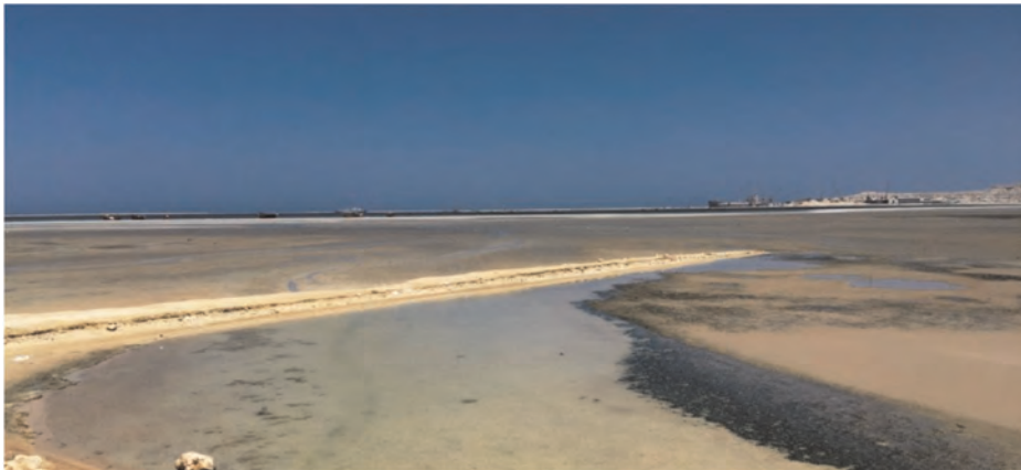
Figure 2. View of the Duqm roads project location showing the extend of muddy sabkha soil.
