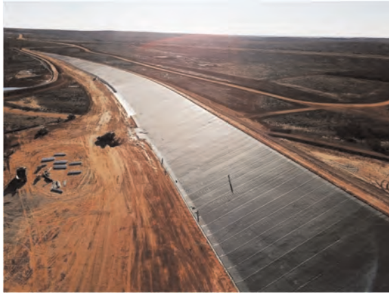
Figure 1. Copper – gold tailings storage facility TSF in South Australia during construction. Note the straight panels on the BGM with no thermally induced wrinkles in extreme 45 deg C heat. This BGM is designed to provide embankment sealing and prevention of tailings migration into sensitive environmental lakes downstream.
