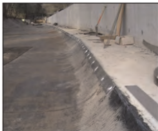
Figure 4. Canal in UK along deep slope.
