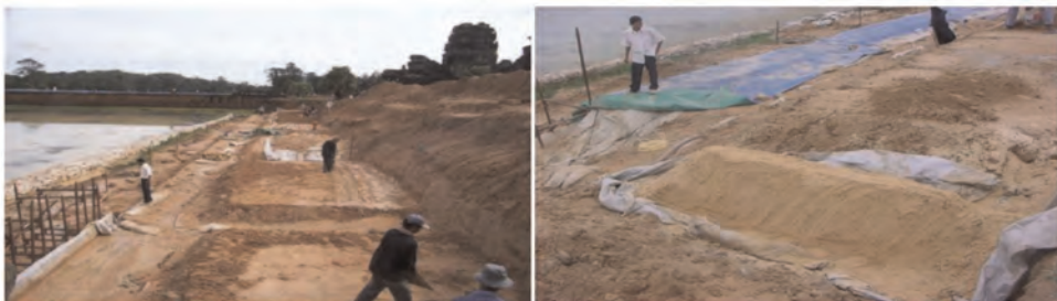
Figure 4. Overview of the working site and detail of the filling of the slurry trench.
