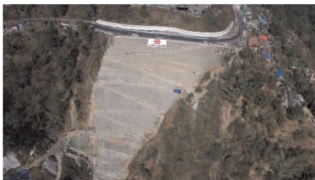
Figure 15. The completed structure.
