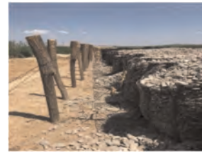
Figure 6. Geomattress filled with a stone material.
