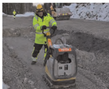
Figure 7. Compaction of the granular material inside the trench.
