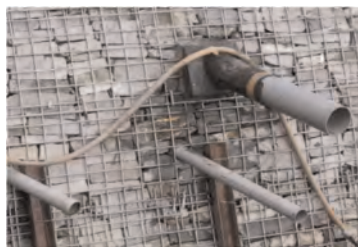
Figure 12. Sub-surface drainage outlets.
