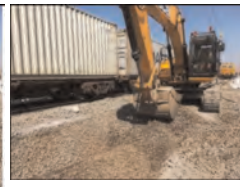
Figure 7. Removal of sub-ballast/blanket.
