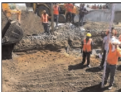
Figure 8. Checking the excavation level.
