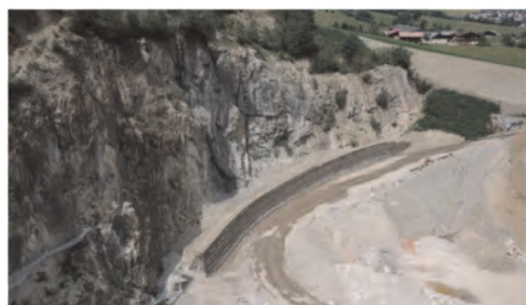
Figure 7. Rockfall protection dam Tenneck.
