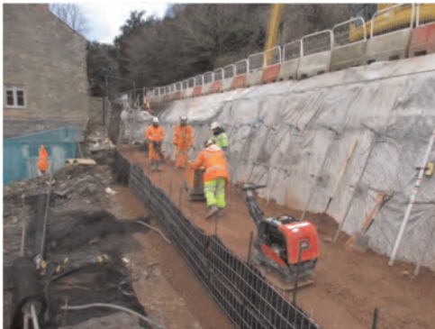
Figure 2. Wall under construction.
