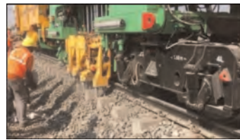
Figure 18(b). Compaction of ballast by dynamic tamping express machine.
