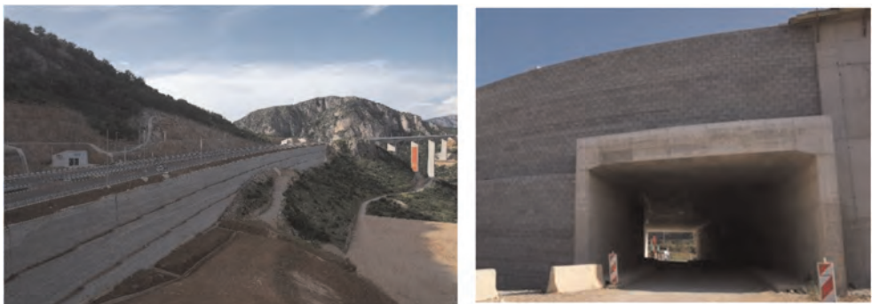
Figure 8. a) Wall with sudden height variation; b) Wall layout around a concrete culvert.
