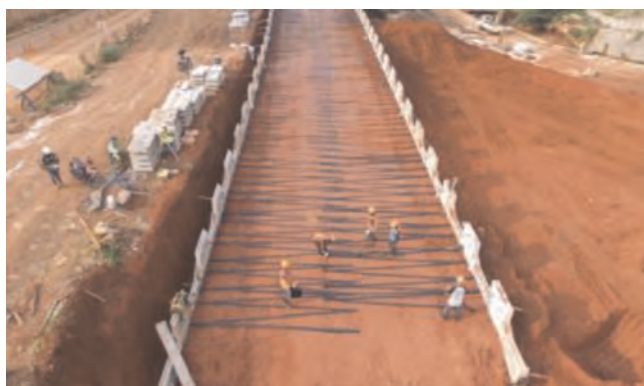
Figure 2. Construction of geoforce segmental retaining wall system.
