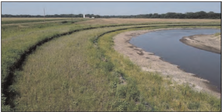
Figure 8. Vegetated SCOURLOK and ARMORMAX performance, July 2021.
