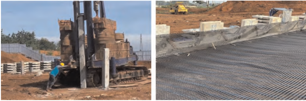
Figure 3. Geosynthetics reinforcement scheme in piled embankment system.
