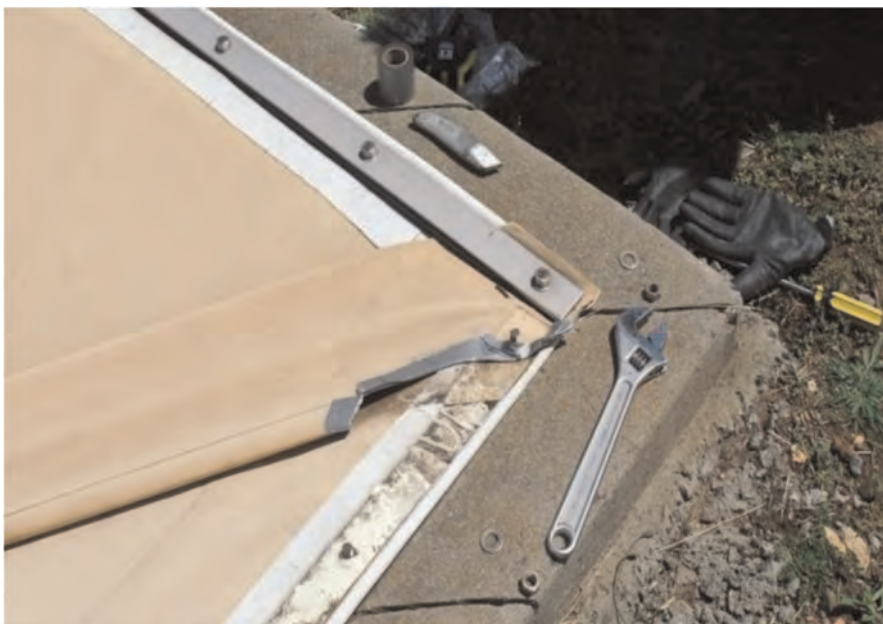
Figure 1. A small cover material sample taken from a ballast tube partly under a batten bar.
