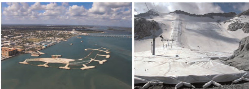
Figure 5. Examples of living breakwaters with geosynthetic (from Phillips, 2013) and of geotextiles for protecting glaciers.
