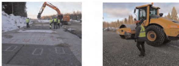
Figure 2. Installed geosynthetic samples for reinforcement/stabilisation function. Compaction of base layer.
