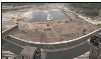
Figure 8. Execution of multistage secondary apron (Kapadia 2020).
