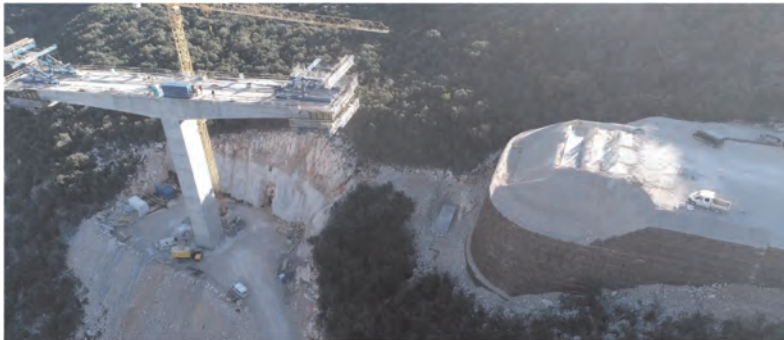
Figure 7. Aerial drone view of the U4 wing wall and abutment of the Dumanja Jaruga viaduct made with the reinforced soil technique with mono-oriented extruded geogrids in HDPE.
