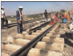
Figure 4. Removing rails.
