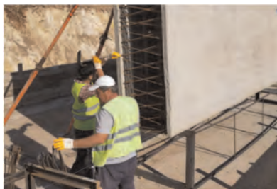
Figure 4c. Installation of horizontal continuity reinforcements.
