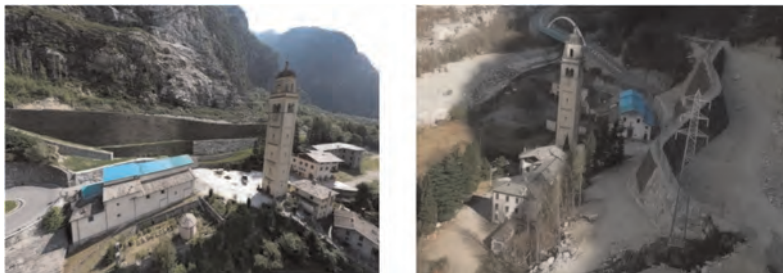
Figure 6. Aerial views of the finished works.
