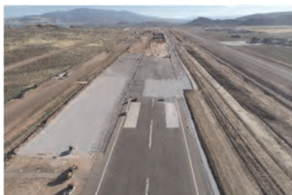
Figure 4a. General view of the site.
