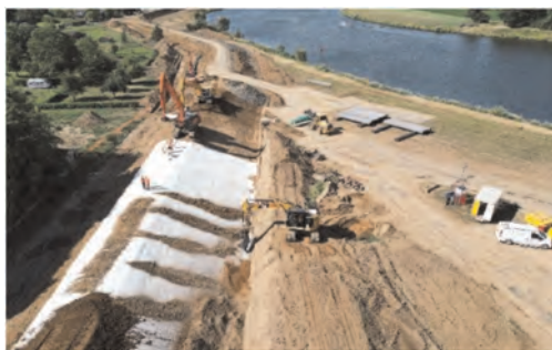
Figure 11. Installation Geosynthetic Clay Liner (GCL) on a levee reinforcement to replace a 1 meter thick clay layer (Beesel Netherlands).
