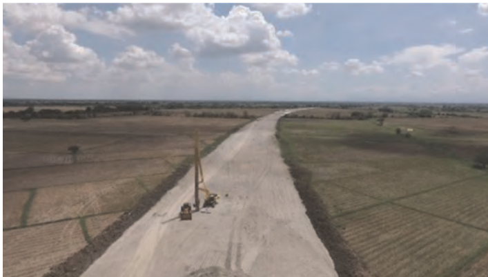
Figure 5. PET high strength geotextile reinforcements laid with principal strength direction across the embankment, followed by placement of gravel layer on top.
