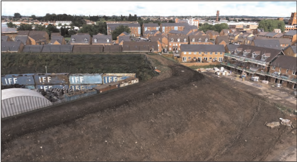
Figure 4. Aerial shot of the completed bund.
