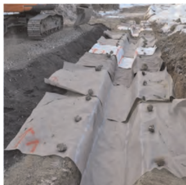
Figure 5. Installed geotextile samples.
