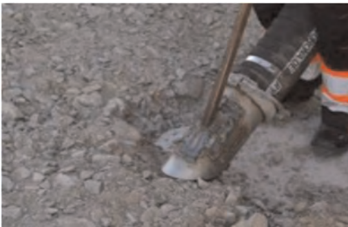
Figure 4. Removing soil with the vacuum / sucking lorry.
