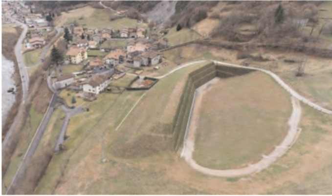
Figure 7. The avalanche dam at the end of construction.
