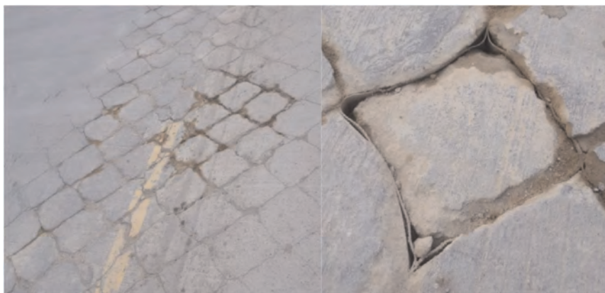
Figure 6. Fail presented in a soft soil with high fines and water presence.
