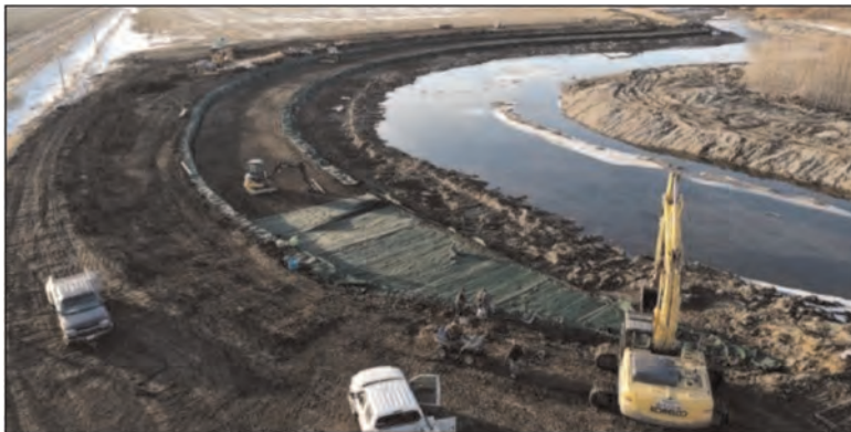
Figure 7. Installation of SCOURLOK and ARMORMAX, January 2021.
