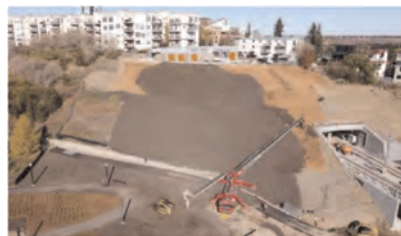
Figure 7. Filling of geocell.
