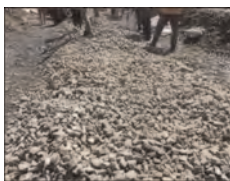
Figure 15. Laying ballast over the blanket layer.
