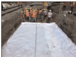
Figure 9. Laying the nonwoven geotextile.
