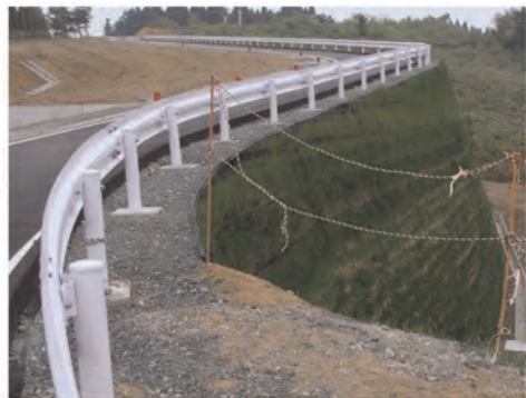
(b) Greened wall facing
