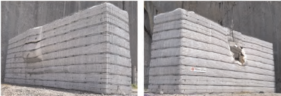
Figure 2. The deformed shape of the embankment after the 5 000 kJ impact.
