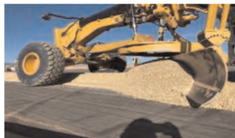
Figure 4b. Equipment and material over BGM.
