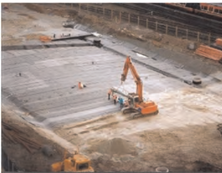
Figure 8a. Membrane installation.
