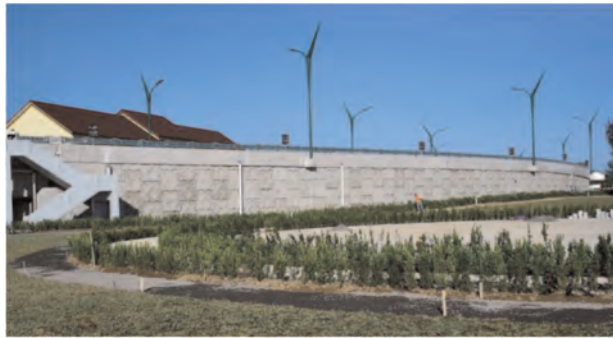
Figure 1. Kretek II Flyover's, Yogyakarta, Indonesia.
