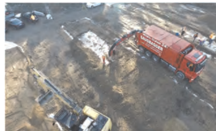
Figure 5. Removal of fill material with a mobile suction excavator.
