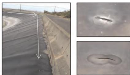
Figure 2. Crest zone of the Buen Paso reservoir, where the geomembrane changes direction and cracks are detected, and examples of cracks.
