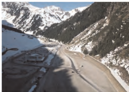
Figure 6. Rockfall protection dam Eisgratbahn-Stubaital.
