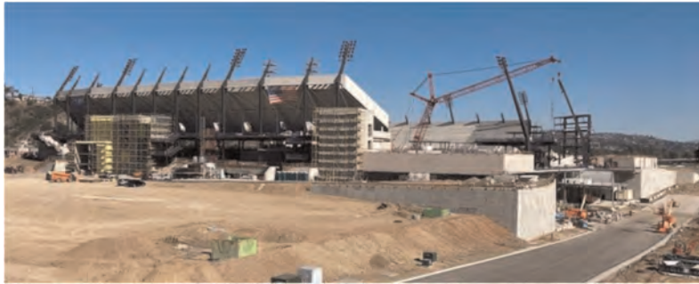
Figure 5. SDSU Stadium under construction.
