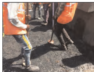
Figure 14. Watering and compaction of infill.
