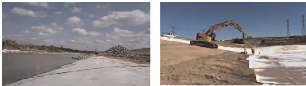
Figure 2. Fully hydrated and/or stubborn groundwater GCL applications in Dyke and/or Canal and/or Pond Applications. Double nonwoven scrim-reinforced GCL being deployed. These GCLs are more robust to installation stresses, have a higher peel than other low grade standard GCLs, and are more weather resistant.
