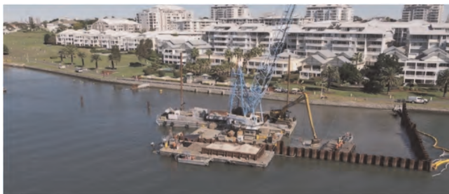
Figure 3. Site remediation in front of modern housing estate (Courtesy of HUESKER Australia).
