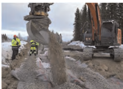
Figure 6. Filling of the trench with granular material.
