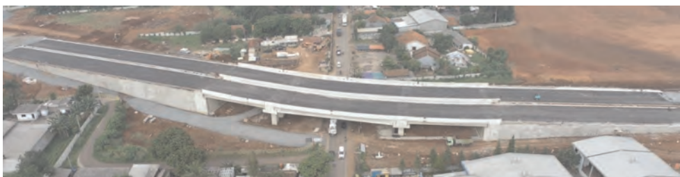
Figure 1. Kadusirung Flyover, Banten, Indonesia.
