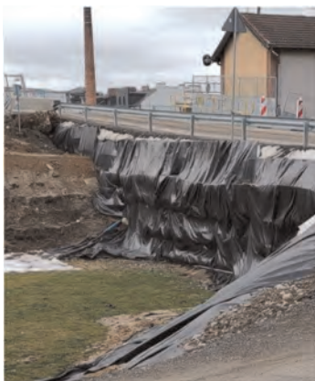
Figure 8. Bypass temporary construction – facing.
