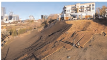
Figure 6. Installation of geocell.
