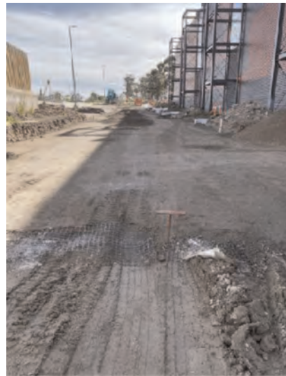
Figure 4. Final pavement ready for asphalt wearing course.
