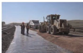
Figure 6b. Sub ballast placement directly on BGM.
