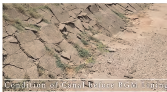
Figure 2. Original condition of canal stretch.
