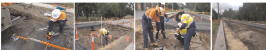
Figure 2. Subgrade preparation and testing.
