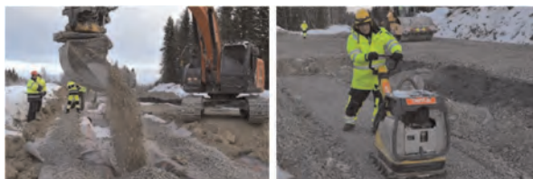
Figure 4. Filtration trench: Backfilling and compaction of upper layer.
