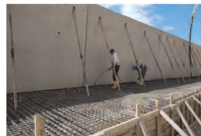
Figure 4d. Pouring of concrete.
