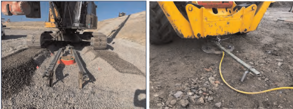
Figure 5. Left: Sand Diego USA 2022 PLT test; Right: Great Yarmouth, UK 2022 PLT.
