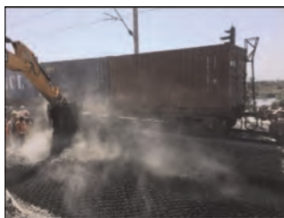
Figure 13. Infilling the geocells.
