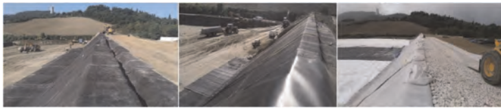
Figure 6. Slopes covered, from left to right, with the rough GCL, the HDP liner, drainage geocomposite (slopes) and nonwoven geotextile (bottom).
