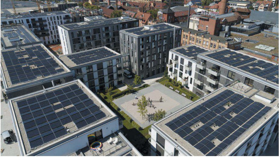
Figure 9.4: Solar panels on the roof of building blocks B (“Bèla”, front) and C (“Citadis”, back). (Source: Maximilian Kamps, Agentur Blumberg GmbH)
