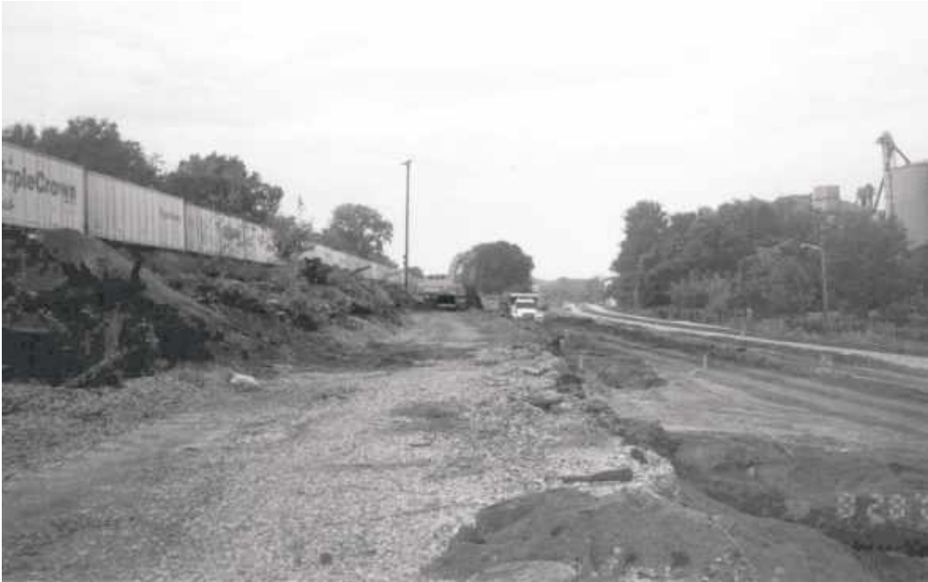
Figure 8-13. The site for mass excavation of a side slope in a rail yard incorporating a track excavator and dump trucks.
