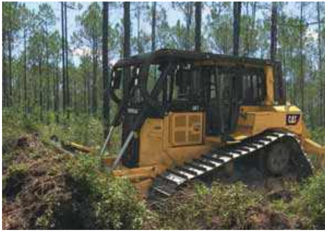
Figure 8-2. Dozer with root rake blade.
