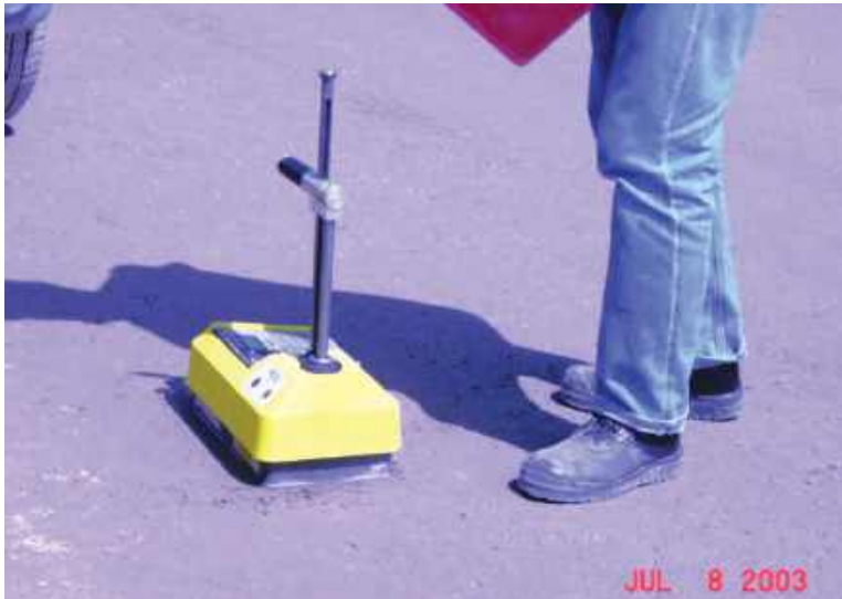
Figure 6-23. Measuring compacted soil density with a nuclear gauge. These devices can measure asphalt density as well as the soil moisture content. The project specifications will direct the required frequency of density testing, often per lift or per volume of compacted soil.
