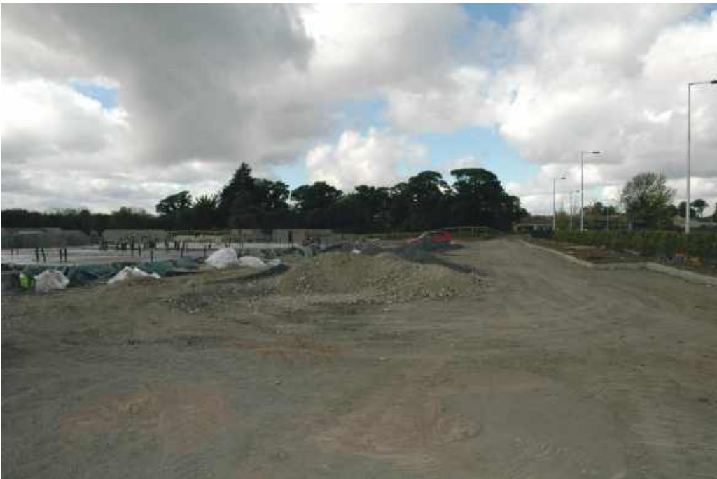
Figure 4-10. Temporary construction road layout built on the location of the future permanent roads.
