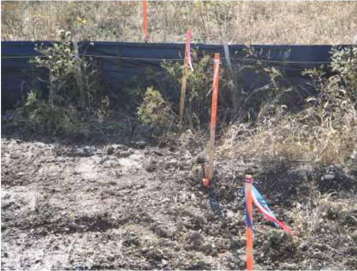
Figure 5-8. Survey staking ribbon color codes.
