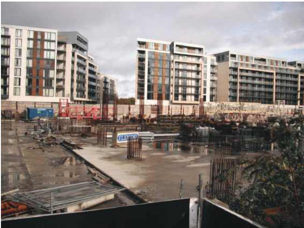
Figure 4-17. A building site during construction.
