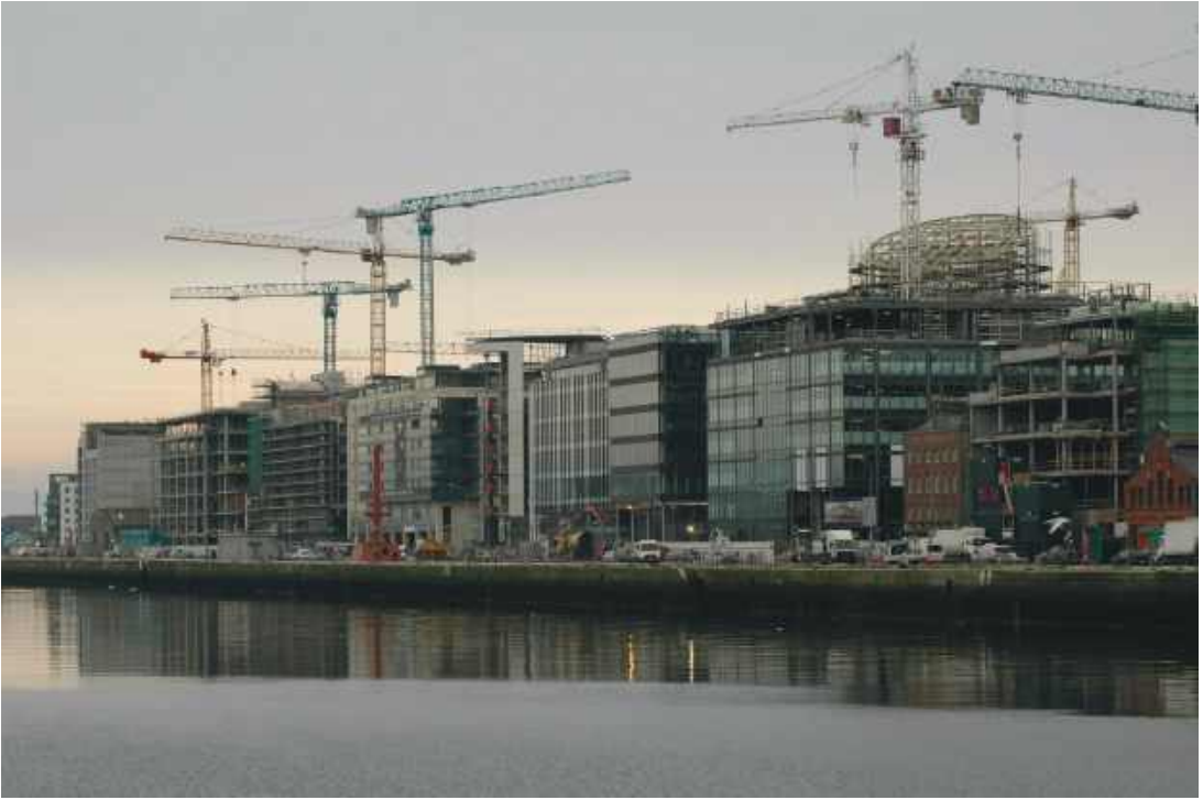
Figure 4-14. The building site during construction.
