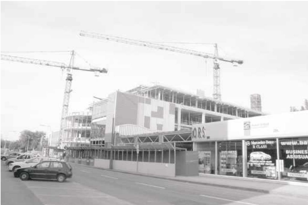
Figure 4-6. Typical hoarding: A solid perimeter barrier on a construction site in Ireland.
