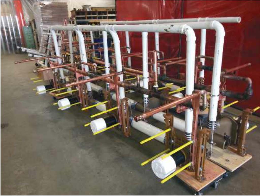
Figure 7-17. Prefabrication of commercial bathroom piping and supports.
