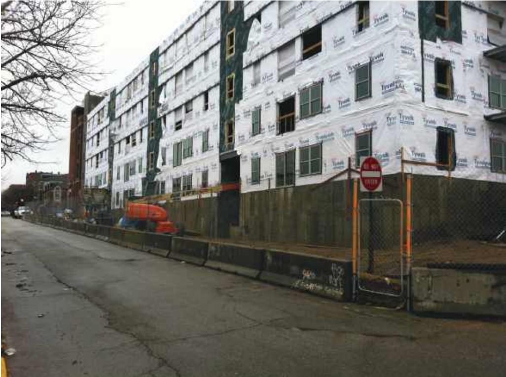
Figure 4-7. Typical fencing with concrete traffic bollards on a construction site in the United States.
