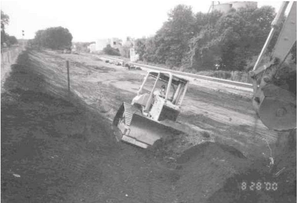
Figure 8-17. Dozer fine grading slope.
