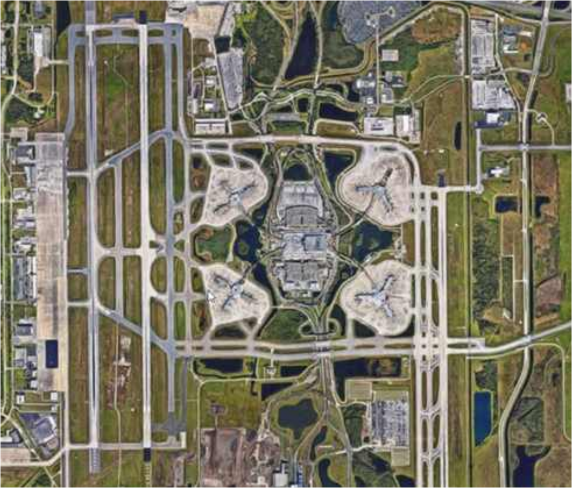
Figure 3-11. Aerial photo of Orlando International Airport (MCO), Orlando, FL (Source: Google Maps).
