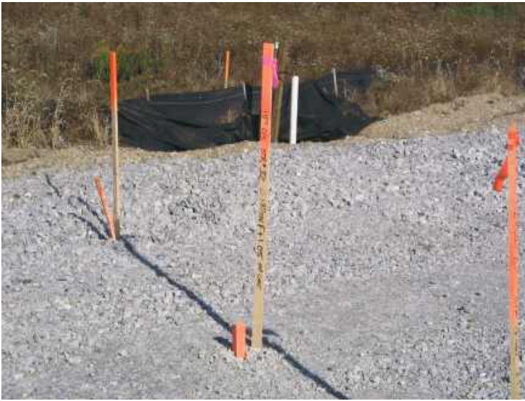
Figure 5-6. Drainage structure grade stake information to 0.01 ft.
