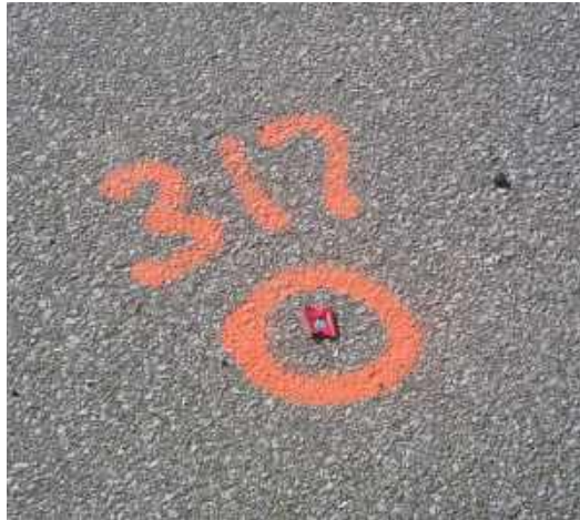
Figure 5-5. Contractor secondary control.
