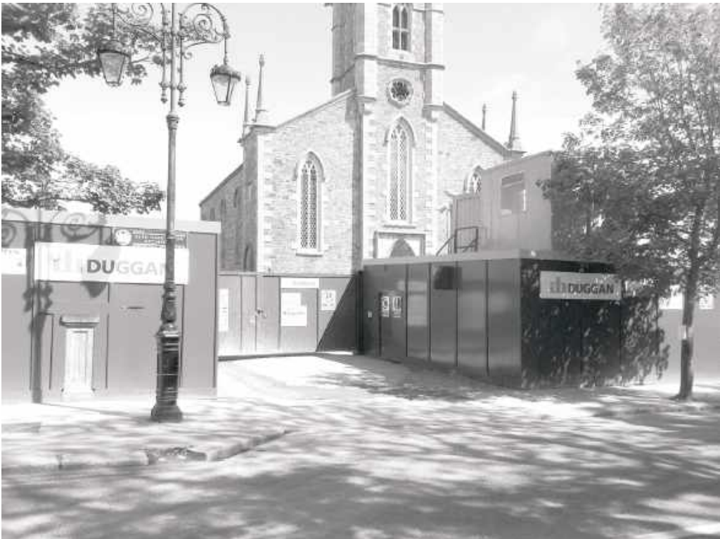
Figure 4-9. What site access is available into the construction site? Is there a clear view for drivers? Is the gate wide enough to take the deliveries expected during construction?
