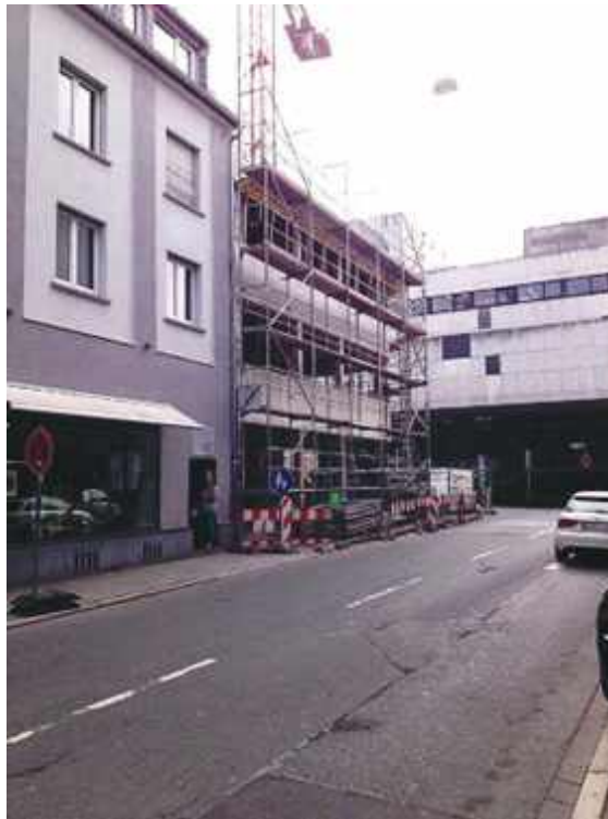
Figure 3-17. Restricted construction site in Darmstadt, Germany.
