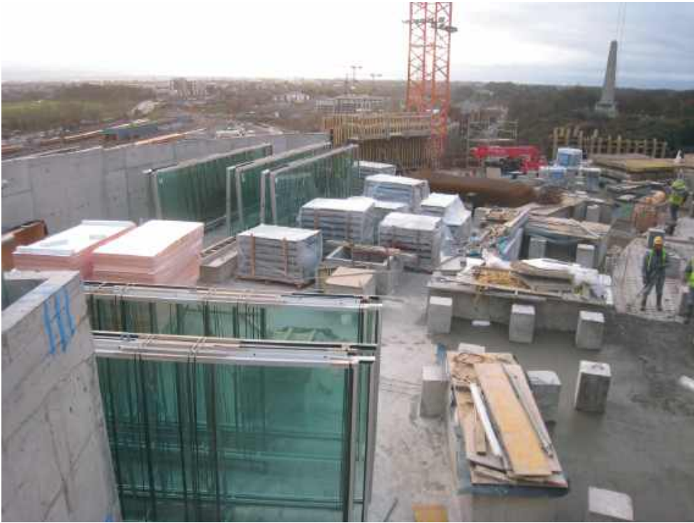
Figure 4-16. Typical site material storage and layout on an Irish construction site.
