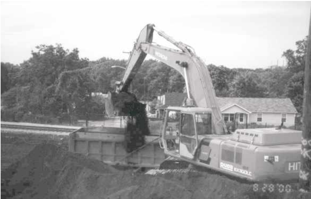
Figure 8-14. Track excavator loading trucks.
