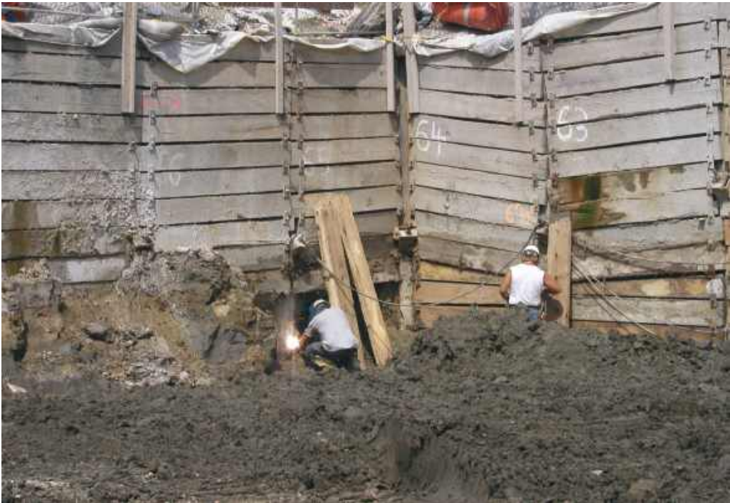
Figure 6-16. Welding bolts to hold wood lagging tightly to the driven H-piles. Encountering a layer of uncommonly plastic soil permits loads from the soil above to induce higher lateral pressures against the excavation supporting structure. Unexpected groundwater might also induce more pressure by increasing the weight of the soil mass while reducing its shear resistance. Not all subsurface conditions are discovered by common soil exploration procedures so builders must be observant.
