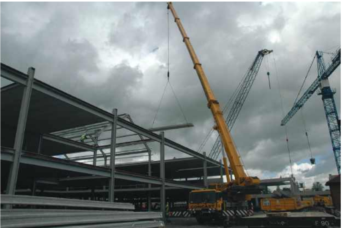
Figure 4-15. Cranage on the building site during construction.
