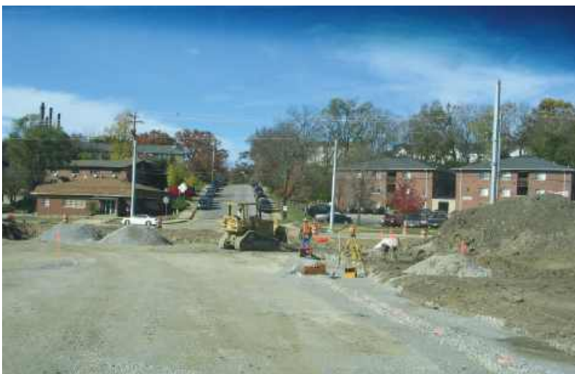
Figure 5-9. Checking grade with laser.
