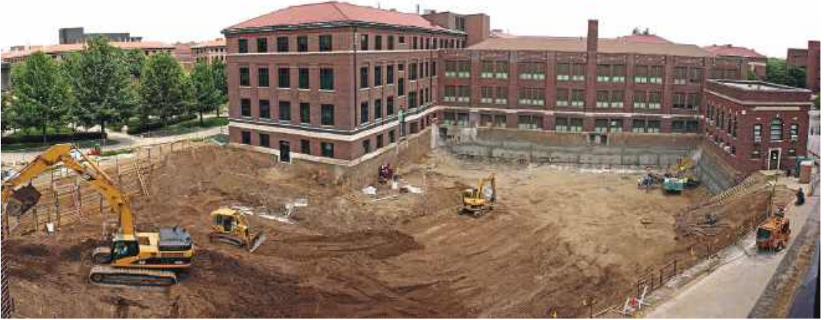
Figure 6-6. Earthwork at a building construction site.
