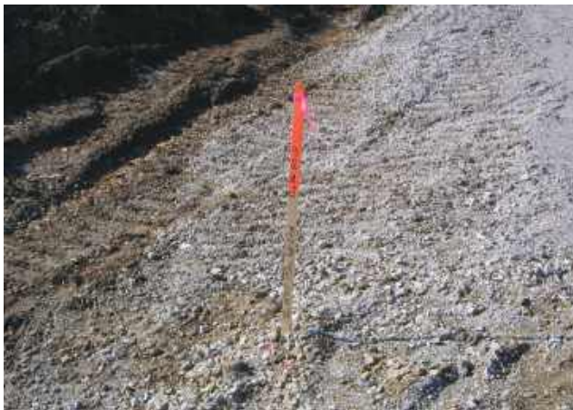
Figure 5-7. Offset stake and color code ribbon.
