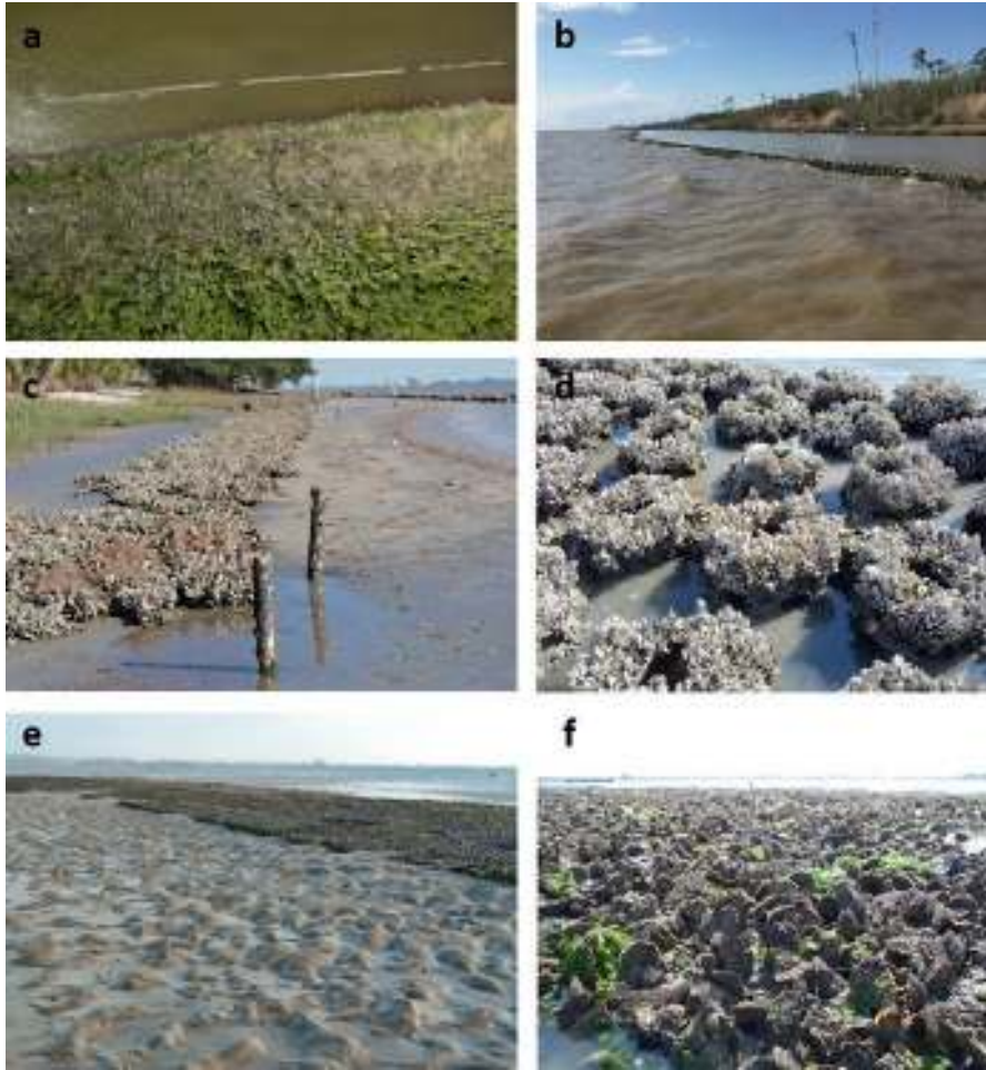
Fig. 13.3 Examples of reefs constructed for shoreline protection and erosion control. (a) Reefs constructed for shoreline protection at Swift Tract Alabama, USA (M-K Brown, TNC); (b) Swift Tract reef demonstrating wave attenuation (M-B Charles, TNC); (c) Reef grown on concrete domes for shoreline protection, Tampa Bay, Florida, USA (B. Hancock, TNC); (d) Concrete domes with 3 years of oyster growth, Tampa Bay, FL, USA (B. Hancock, TNC); (e) Reef consisting of gabions filled with oyster shells constructed for erosion control of an intertidal mudflat of Viane, Oosterschelde, The Netherlands (T. Ysebaert, WMR); (f) Reef at Viane after 3 years of oyster growth, Oosterschelde, The Netherlands (B. Walles, WMR)
