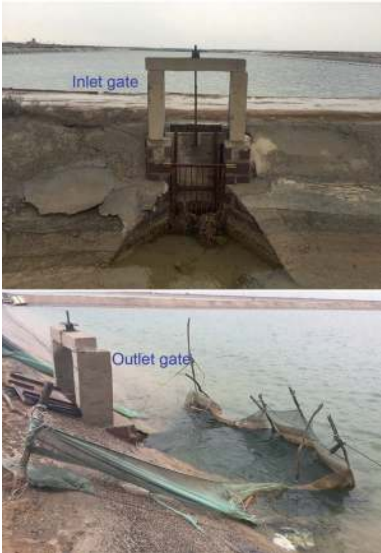
Fig. 4.4 Inlet gate with channel higher than water level; and outlet gate with channel lower than water level. (From Mao)
