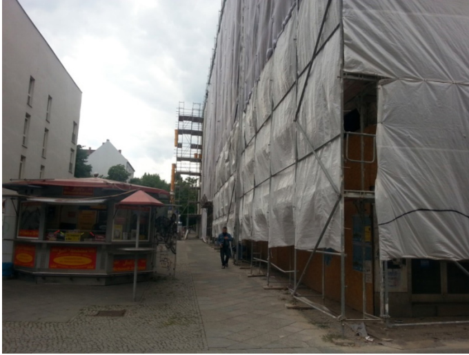
Fig. 32 Building under construction
