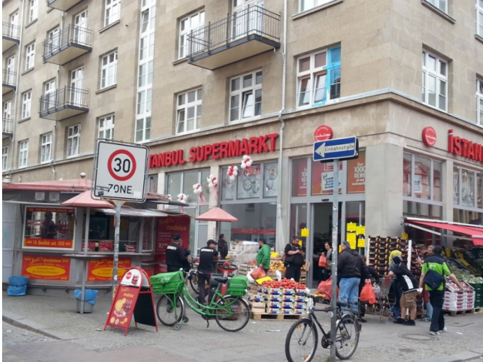
Fig. 33 Upgraded building with new supermarket
