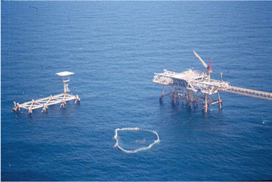
Fig. 13.5 Dunlop Tempest 4 TM 18,000 m 3 cage system in 40 m of water at the platform site 54 km offshore on the central coast of Texas
