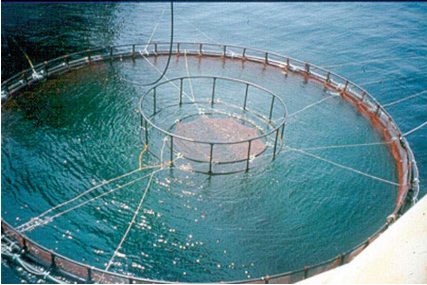
Fig. 13.7 10,000 m 3 double ring HDPE 30 m diameter net pen moored between two platforms off of the central Texas coast
