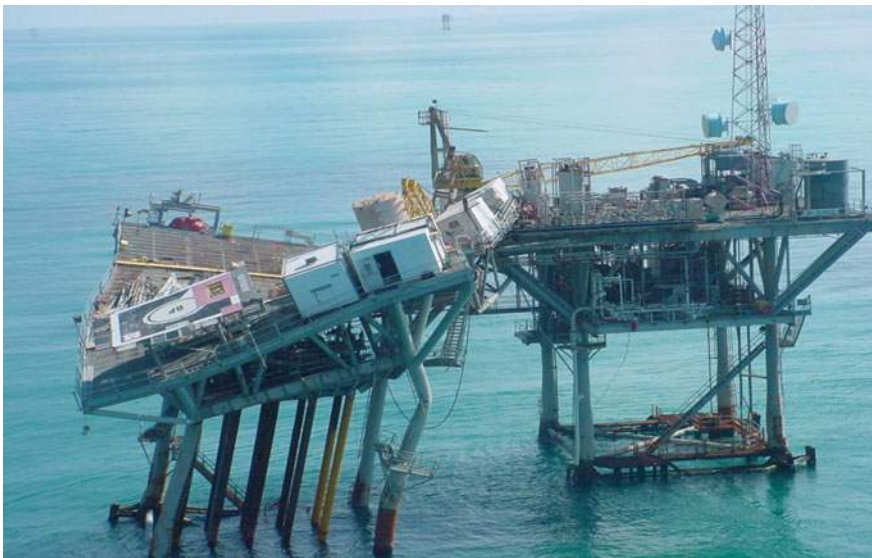
Fig. 13.2 Offshore platform damaged during a hurricane off of Louisiana
