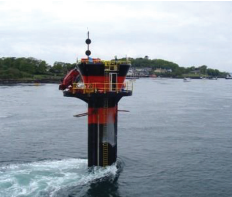
FIGURE 13.7 The world's first commercial scale and grid-connected tidal stream generator—SeaGen—in Strangford Lough. (Adapted from “Tidal power,” Wikipedia, the free encyclopedia, 2013.)
