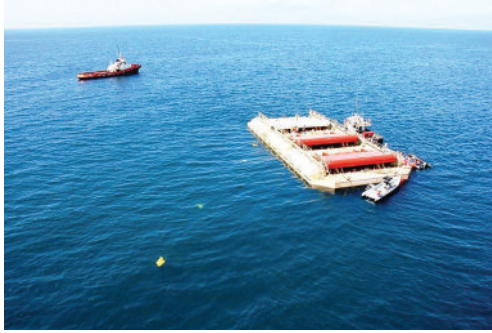
FIGURE 13.3 WaveRoller wave energy farm installation in Peniche, Portugal. (Adapted from “Wave power,” Wikipedia, the free encyclopedia, 2013.)
