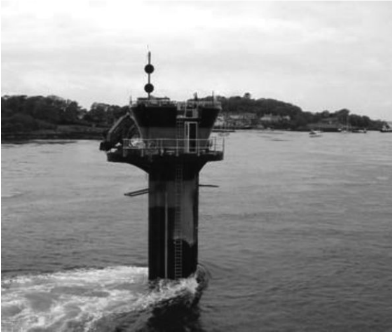
FIGURE 13.7 (See color insert.) The world's first commercial scale and grid-connected tidal stream generator—SeaGen—in Strangford Lough. (Adapted from “Tidal power,” Wikipedia, the free encyclopedia, 2013.)
