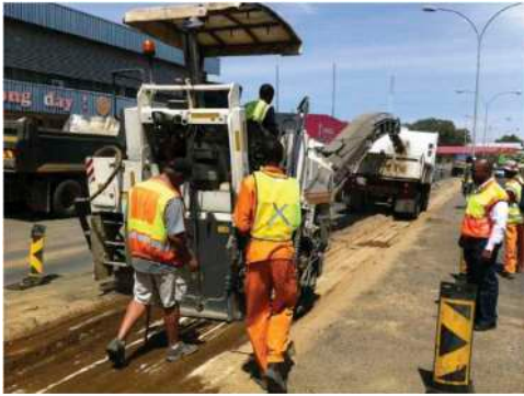
Figure 11. Milling existing asphalt.
