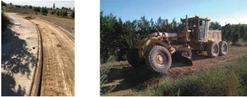
Figure 2. Milling procedure of the original surface and levelling process of the borrow soil.
