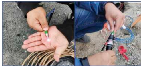
Figure 4. The inspection of the optical fibre sensors.
