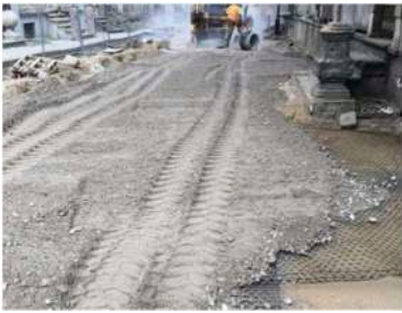
Figure 4. Installation of geogrid.
