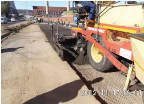
Figure 13. Installation of BSM with paver.
