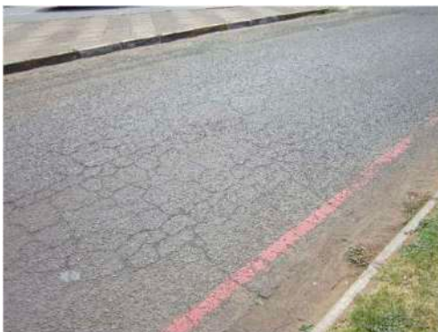
Figure 15. McGregor Street prior to rehabilitation.
