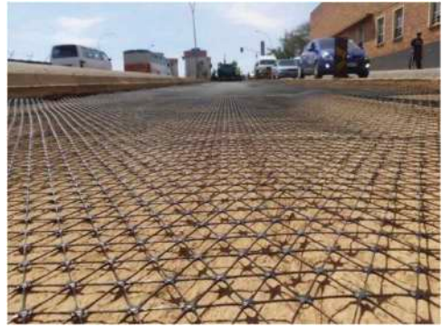
Figure 12. Installation of stabilisation geogrid.
