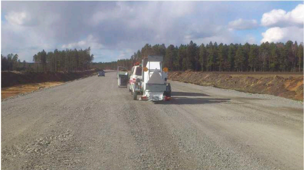
Figure 1. Testing on the subbase in April 2012.
