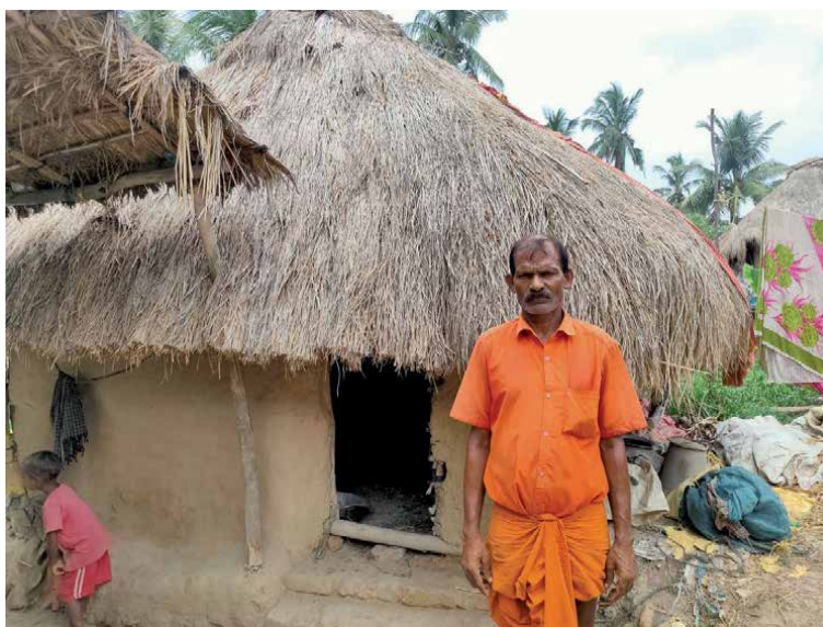
Figure 4. Sheep houses with mud flooring and thatched roof.
