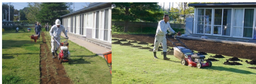
Fig. 17.7 The decontamination experiment conducted on a nursery lawn on the UTokyo Campus (Fukuda et al. 2013a)
